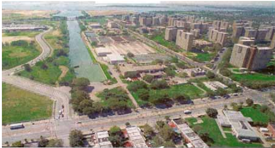
Aerial View of 26th Ward WPCP Photo Courtesy of NYCDEP
