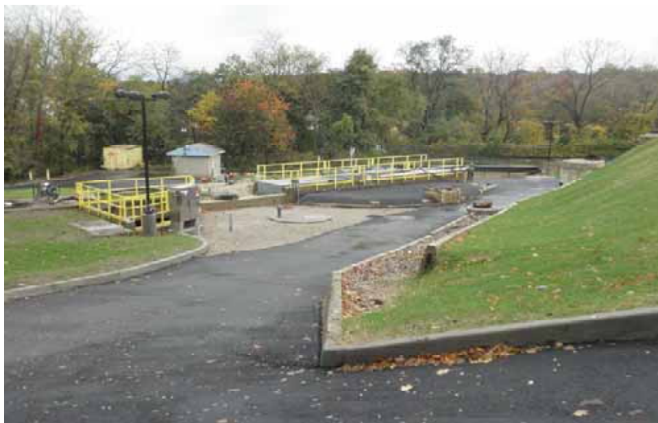
Newly Installed Sequence Batch Reactor Photo Courtesy of SCDPW
