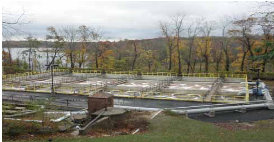
Pre-equalization Tanks with Nissoquogue River in Background Photo Courtesy of SCDPW
