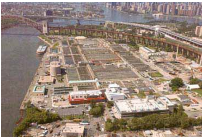
Aerial View of Wards Island WPCP Photo Courtesy of NYCDEP
