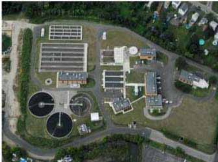
Aerial View of Upgraded Facility Photo Courtesy of Stratford WPCF
