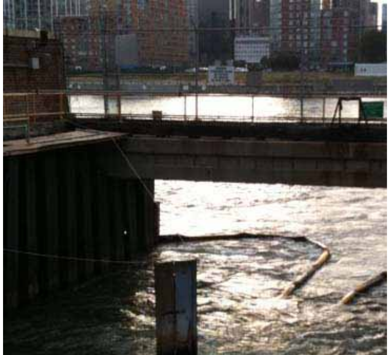
TransCanada Ravenswood Generating Station, July 2010 Photo by E. Powers, IEC
