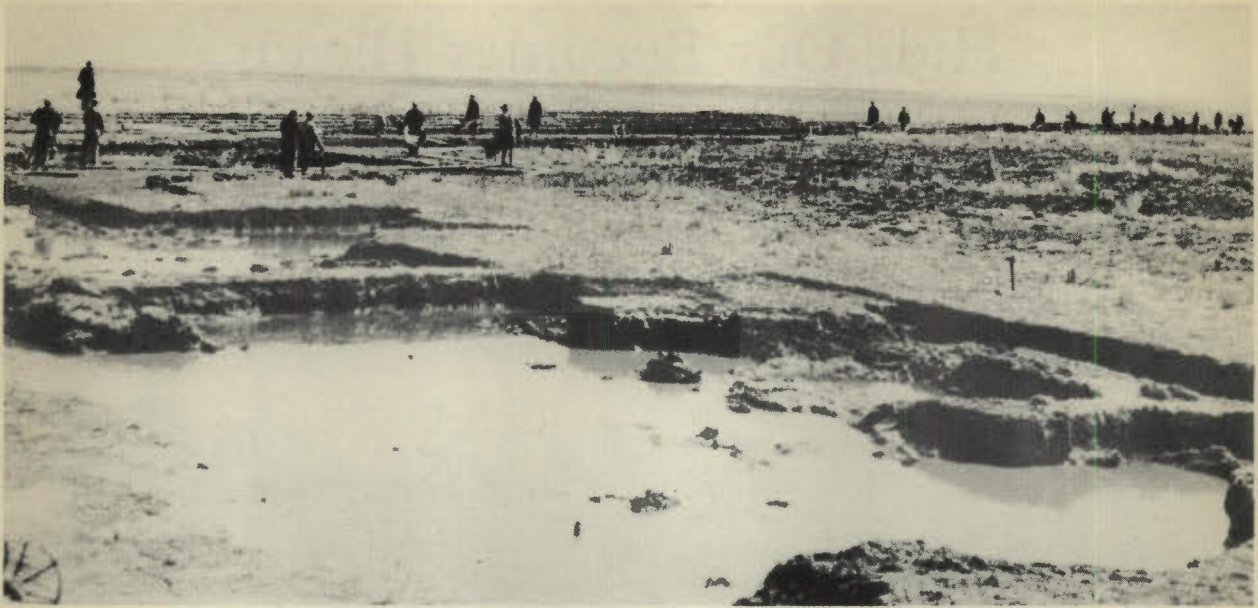
Building the dike to control the flow of water
