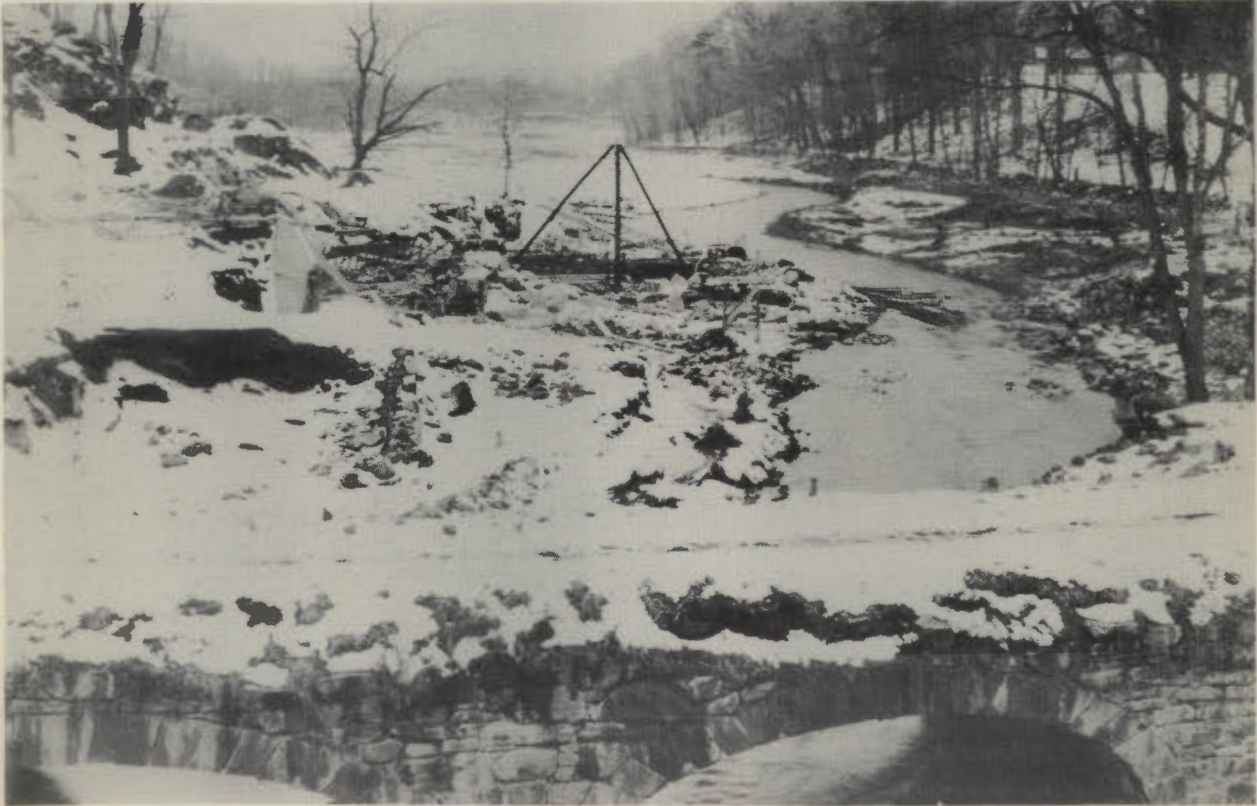
Building the dam at Speedwell Park, Morristown
