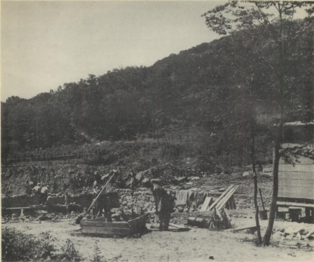
The beginning of the new Administration Building
