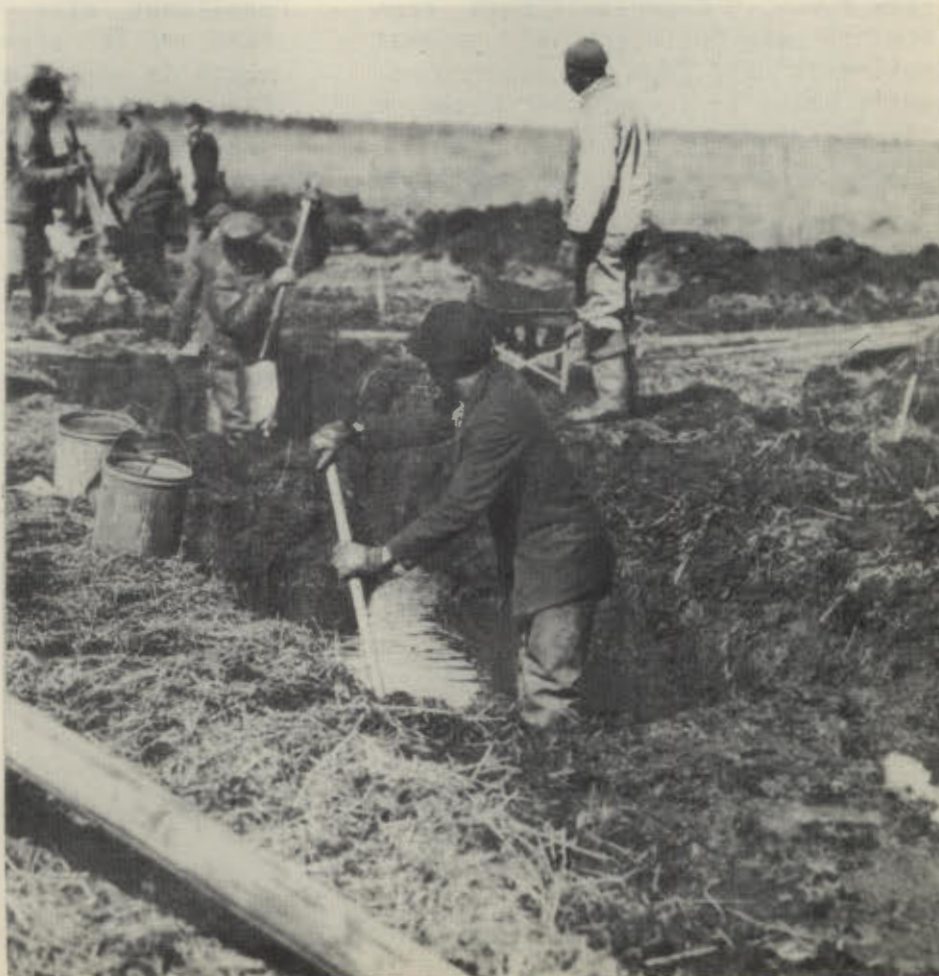
Excavating drainage ditches
