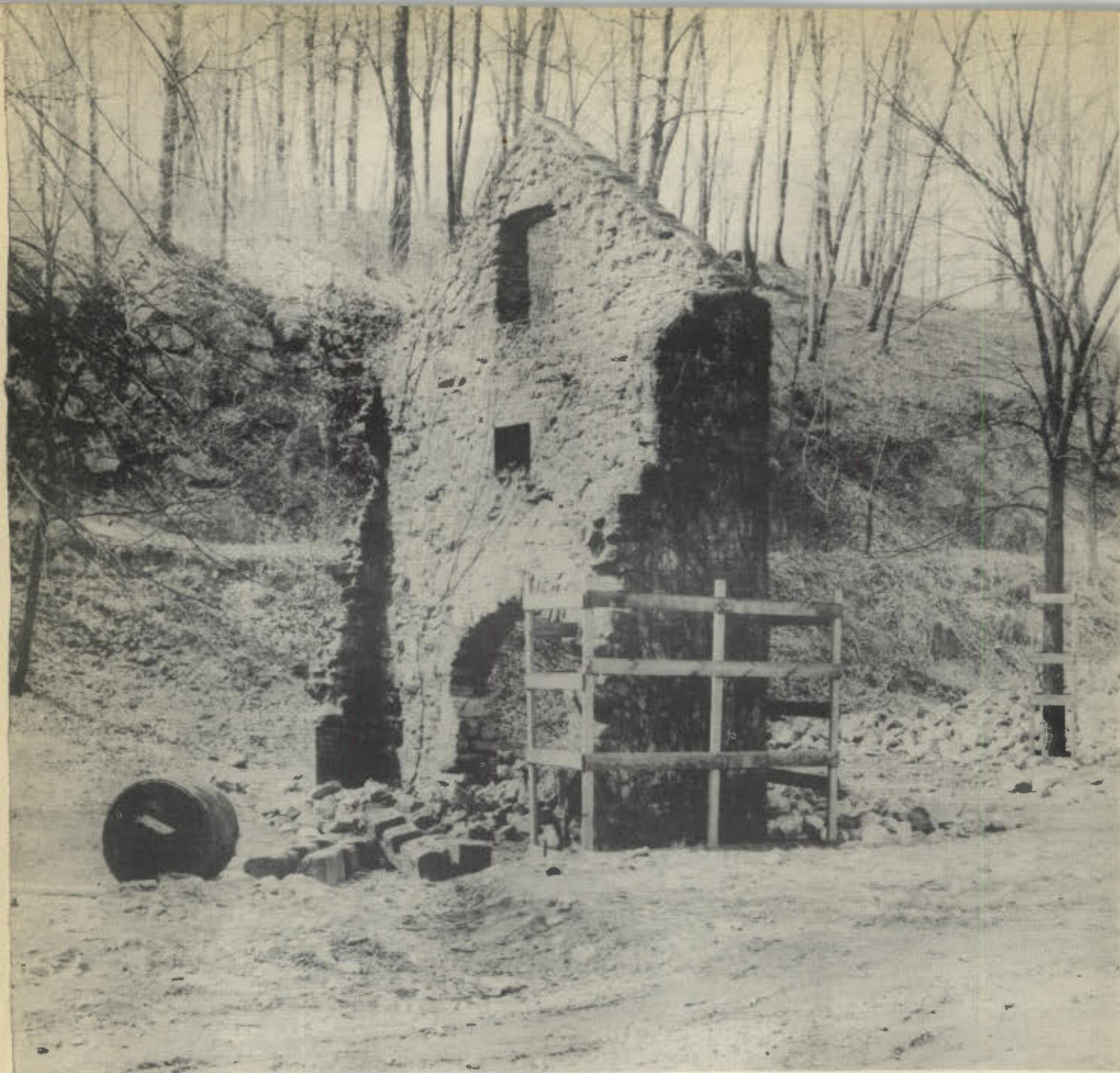
Ruins of the Speedwell Iron Works
