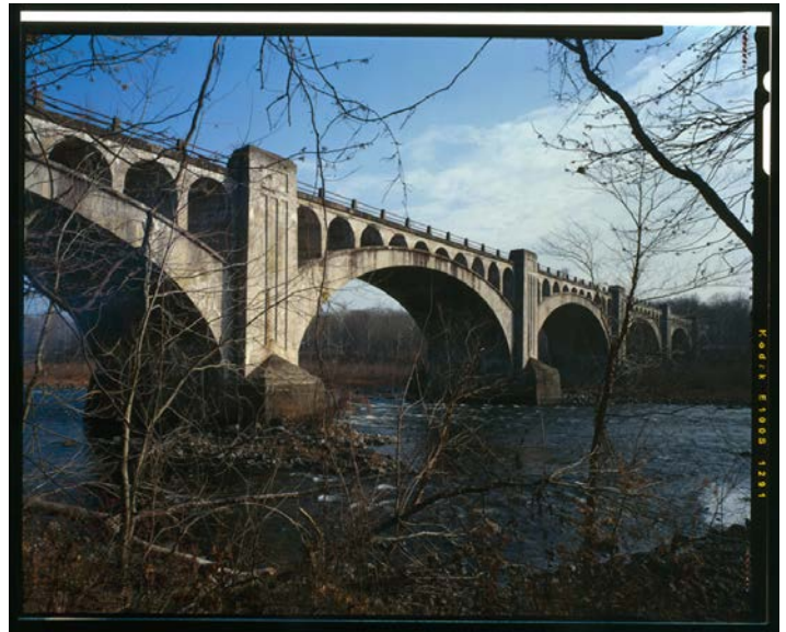
2000 photograph of the Delaware River Viaduct, Knowlton Township, Warren County, NJ and Upper Mount Bethel Township, Northampton County, PA (1911) [Source: Library of Congress, HABS/HAER/HALS Collection].
