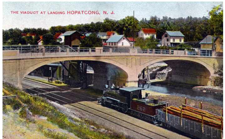
Circa 1910 postcard of Landing Road bridge showing active Morris Canal at right [Source: www.landingnewjersey.com ].
