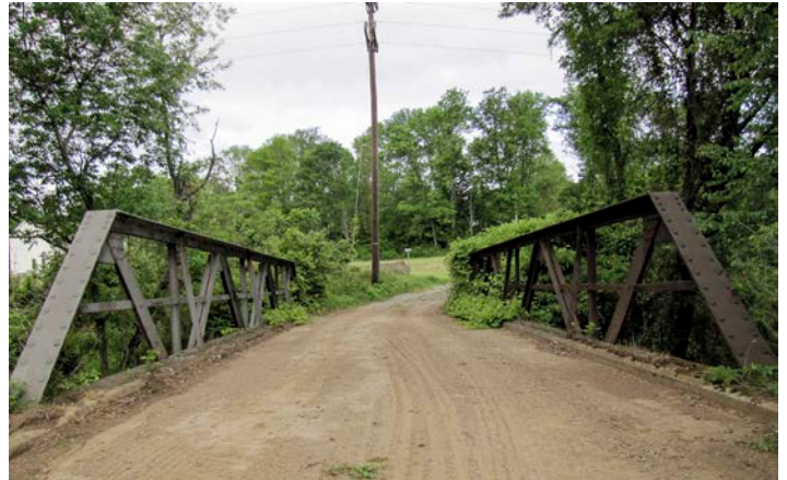
Farm Lane over DL&W (MP 62.39), Mansfield Township, Warren County (1900/1914).
