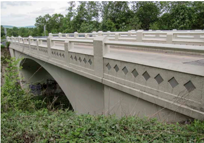
The replacement Hope Road Bridge over DL&W New Jersey Cutoff, constructed 2006.
