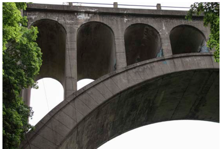
Paulins Kill Viaduct, Knowlton Township, Warren County (1911).
