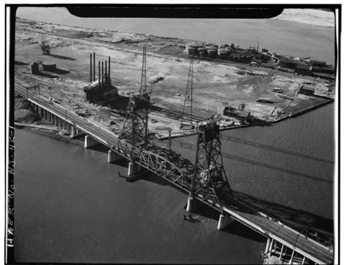
Lower Hack Bridge, Jersey City and Kearny Town, Hudson County, 1928 [Source: Joseph Elliott 2005].
