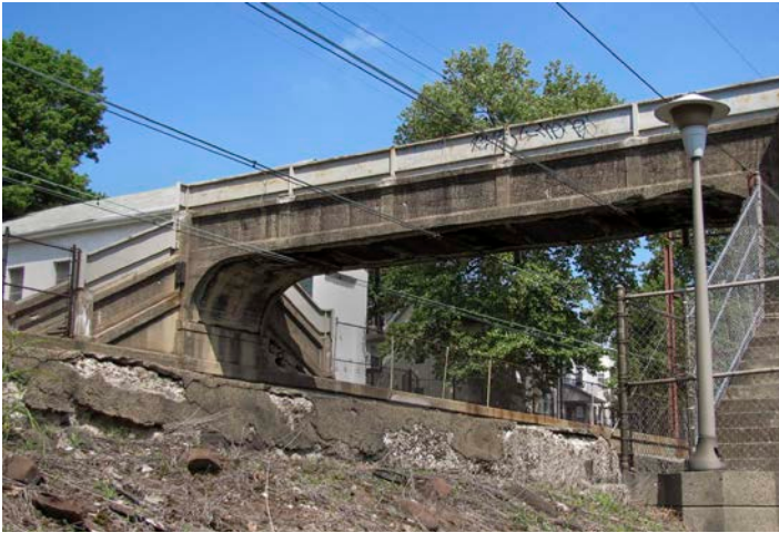
North Maple Avenue Footbridge, East Orange City, Essex County (1923).
