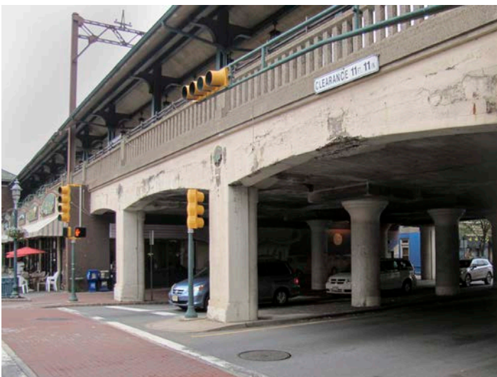
South Orange Station Viaduct, South Orange Village Township, Essex County (1916).
