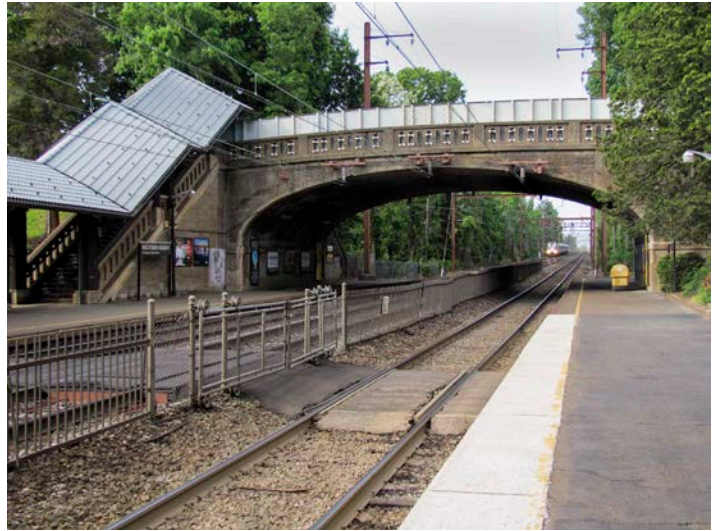
Montrose Avenue over DL&W, South Orange Village Township, Essex County (1917).
