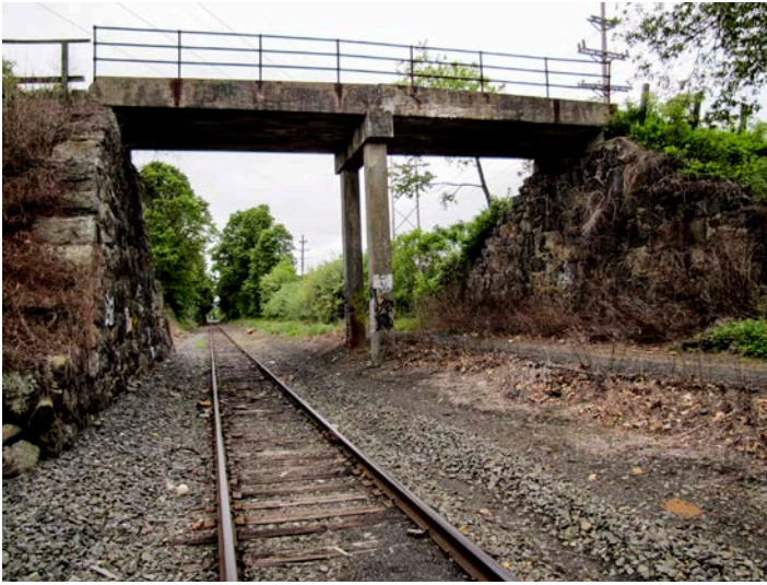
Farm Lane over DL&W (MP 58.61), Mansfield Township, Warren County (1913).
