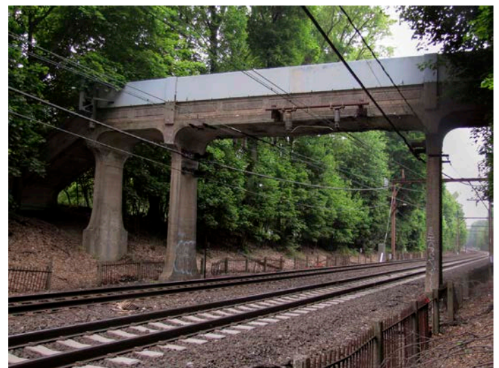
Ridgedale Avenue Footbridge, Madison Borough, Morris County (1916).
