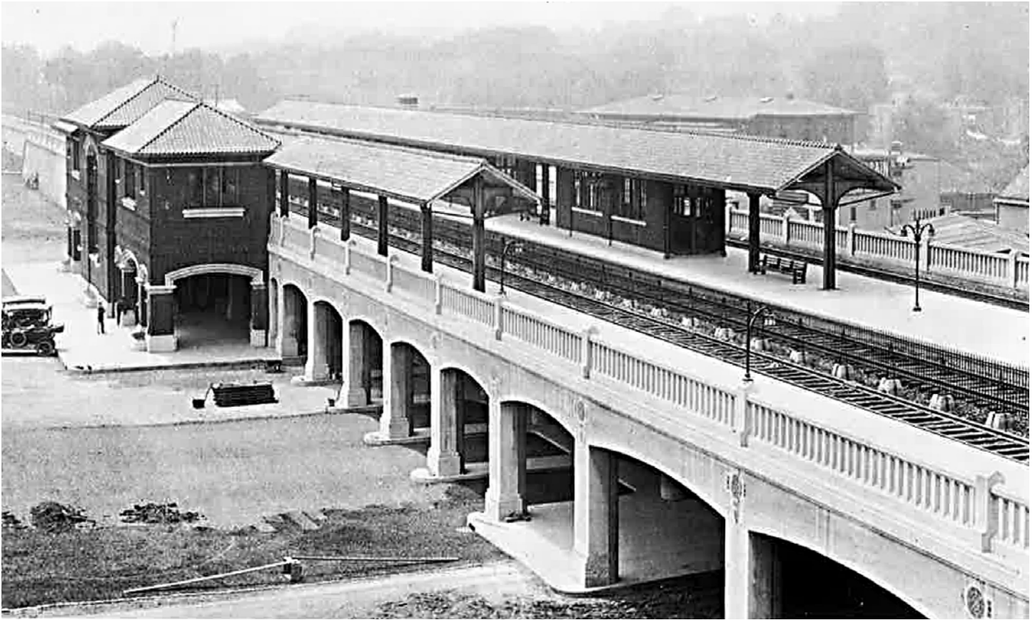
1916 photograph of the South Orange Station Viaduct, South Orange Village Township, Essex County [Source: Taber III 1980].
