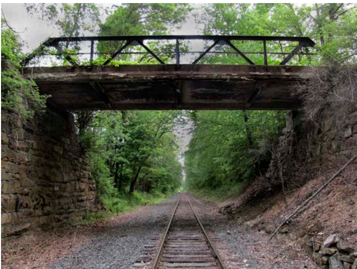
Farm Lane over DL&W (MP 62.39), Mansfield Township, Warren County (1900/1914).
