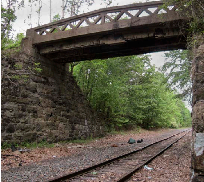
Brickyard Road over DL&W, Mansfield Township, Warren County (1913).
