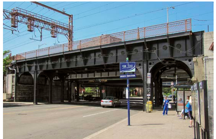
DL&W over Broad Street, City of Newark, Essex County (1903).
