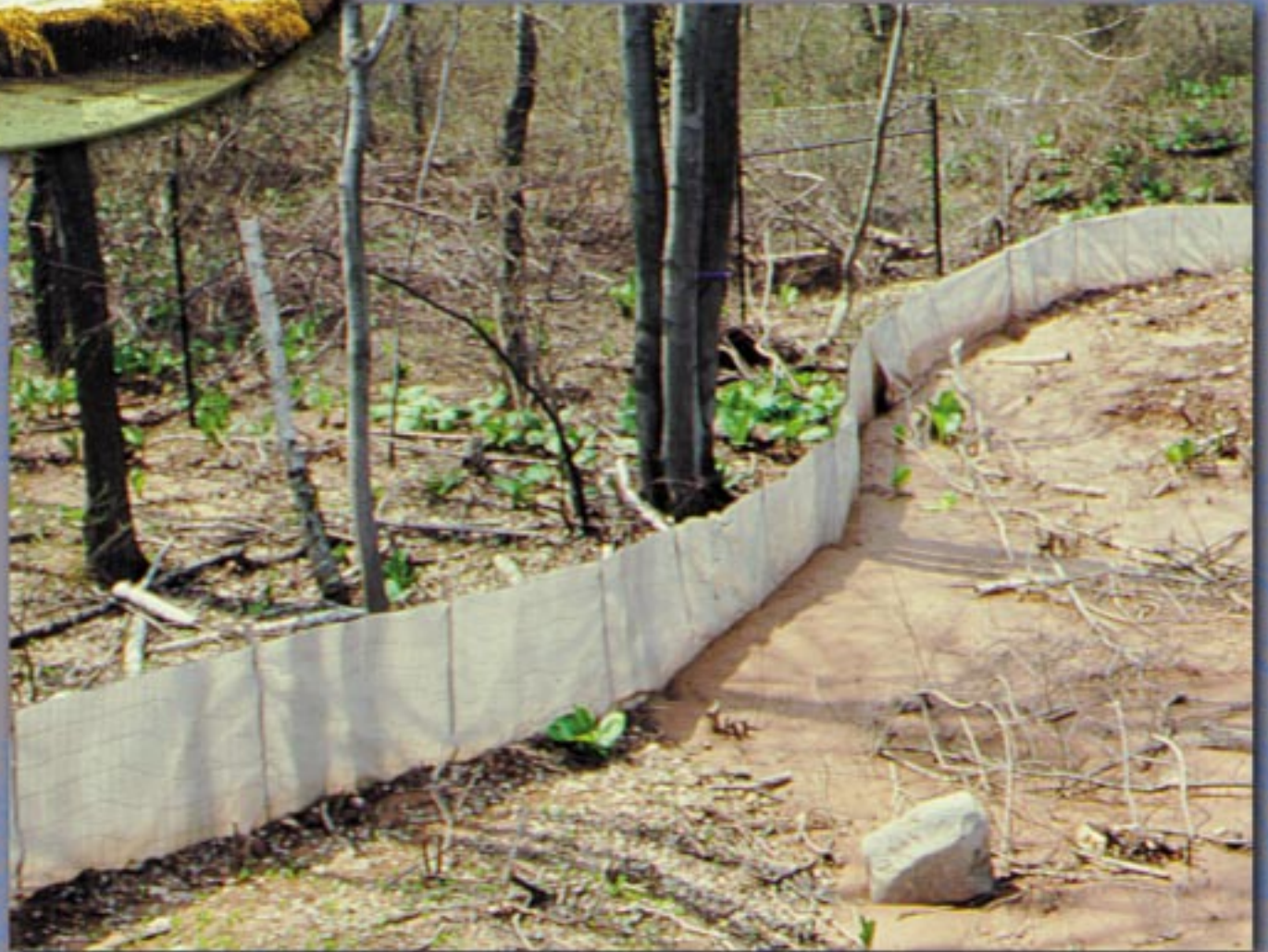
Top: Plastic and hay prevent rain from washing away soil. Right: A silt fence protects a nearby forest from mud.
