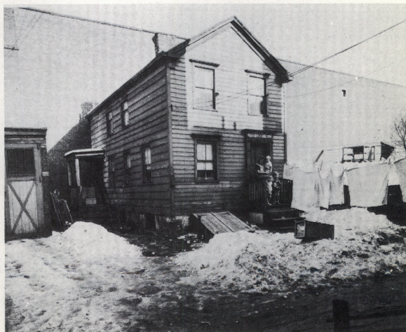
A TYPICAL SLUM-EXTERIOR
