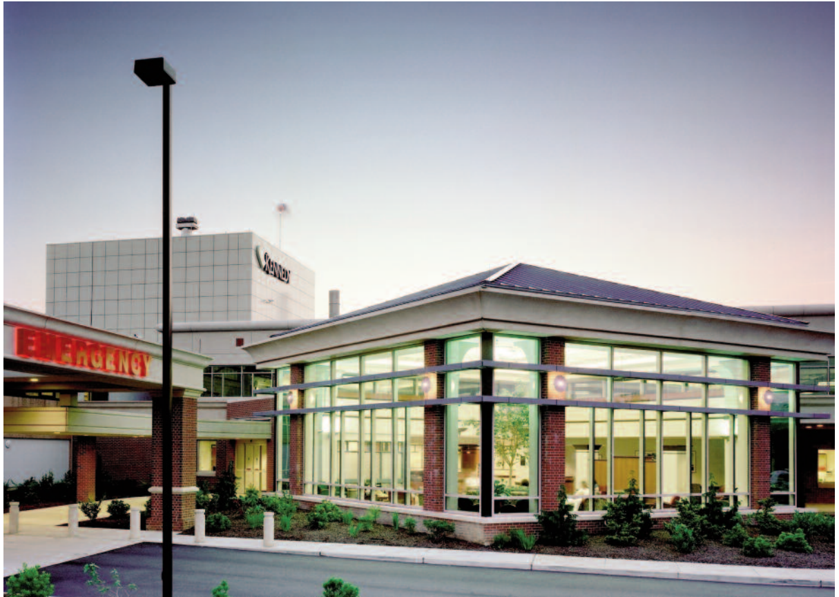
Kennedy University Hospital - Washington Township
