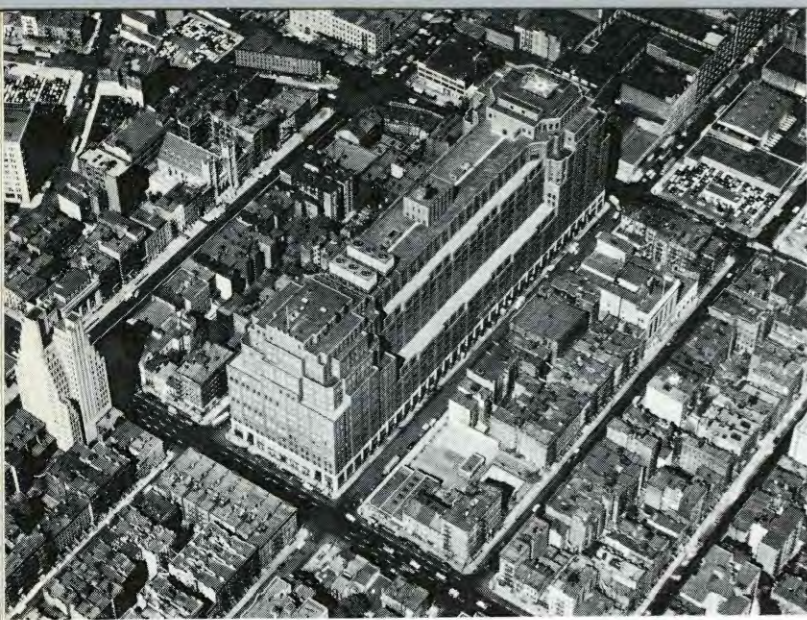
The Port Authority Building, at 15th Street and 8th Avenue in Manhattan, houses the bi-state agency's offices. Its street floor provides off-street truck terminal facilities for consolidating freight shipped on one or more of seven railroads, while its basement is the Railway Express Agency's lower Manhattan base station.
