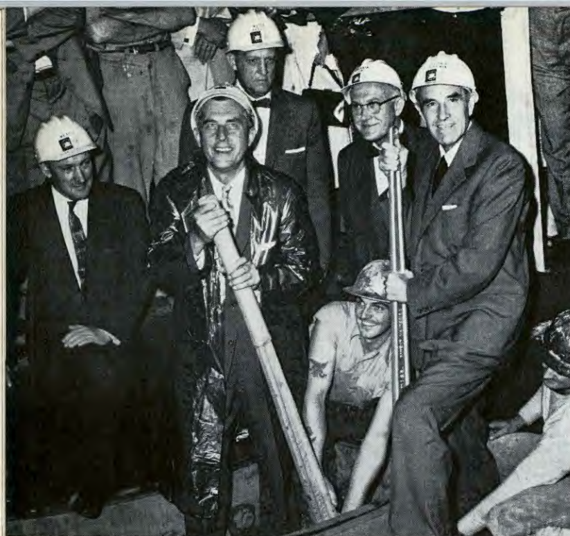
On June 28, 1956, Governor Robert B. Meyner of New Jersey, left, and Governor Averell Harriman of New York tightened the final bolt of Lincoln Tunnel Third Tube's cast iron and steel outer shell, marking completion of compressed-air tunneling operations. Chairman Donald V. Lowe and Chief Engineer John Kyle (far left) watch ceremony at which new bi-state link was heralded.
