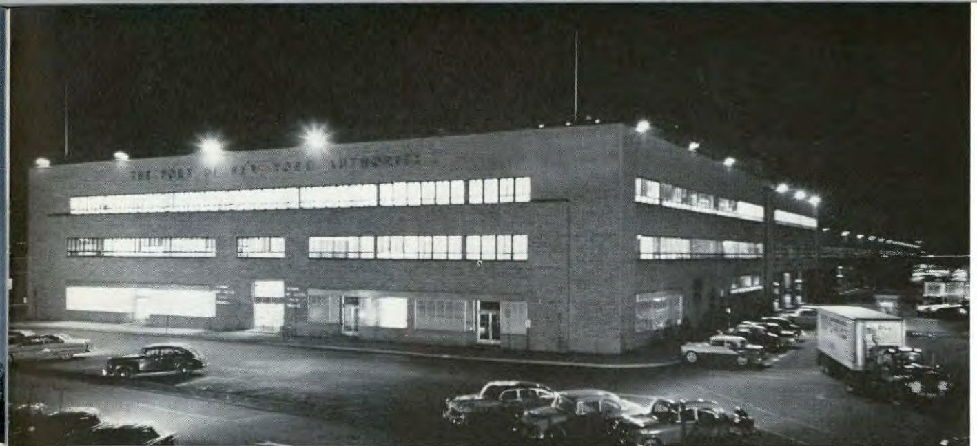
The world's largest truck freight terminal, the Newark Union Motor Truck Terminal, can accommodate 160 trucks at one time.
