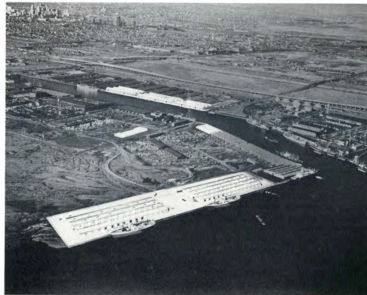
Construction projects under way or planned at Port Newark in 1956 are drawn on this photograph. New structures comprise Norton, Lilly terminal (foreground), new cargo terminal building and a unique bulk wine terminal (on channel's southern shore). On north bank, a three-berth cargo terminal was also under construction.
