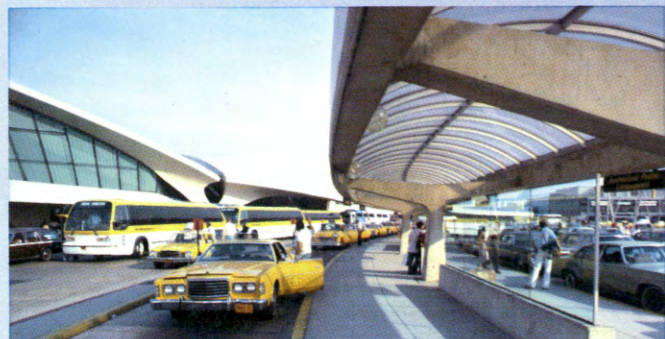
A new canopied frontage at Kennedy International Airport to help reduce traffic congestion in the central terminal area.
