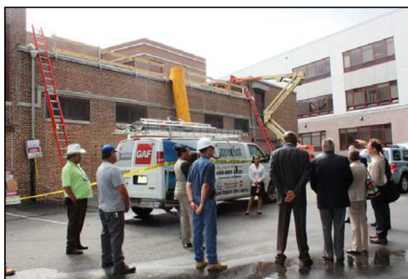
Roof repairs at Madison Avenue School in Irvington
