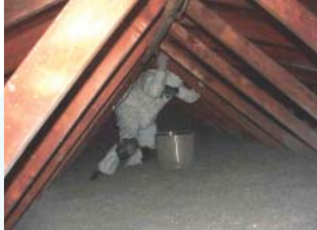
The New Jersey Comfort Partners Program helps seniors and low-income households throughout New Jersey to find ways to reduce their energy usage and improve their overall standard of living by reducing their utility bills. The home pictured above, in Freehold, NJ has achieved heating and air conditioning savings by sealing numerous air leakage sites in the attic and sealing gaps in the ductwork.
