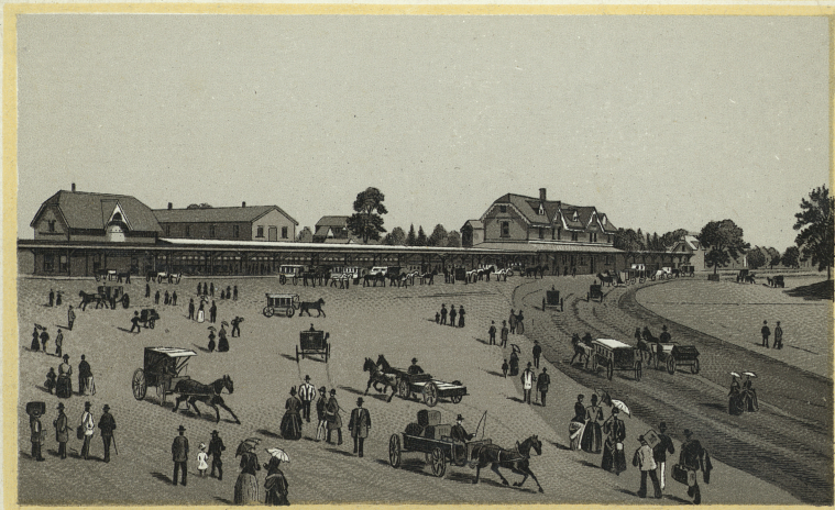
MAIN DEPOT, ASBURY PARK.
