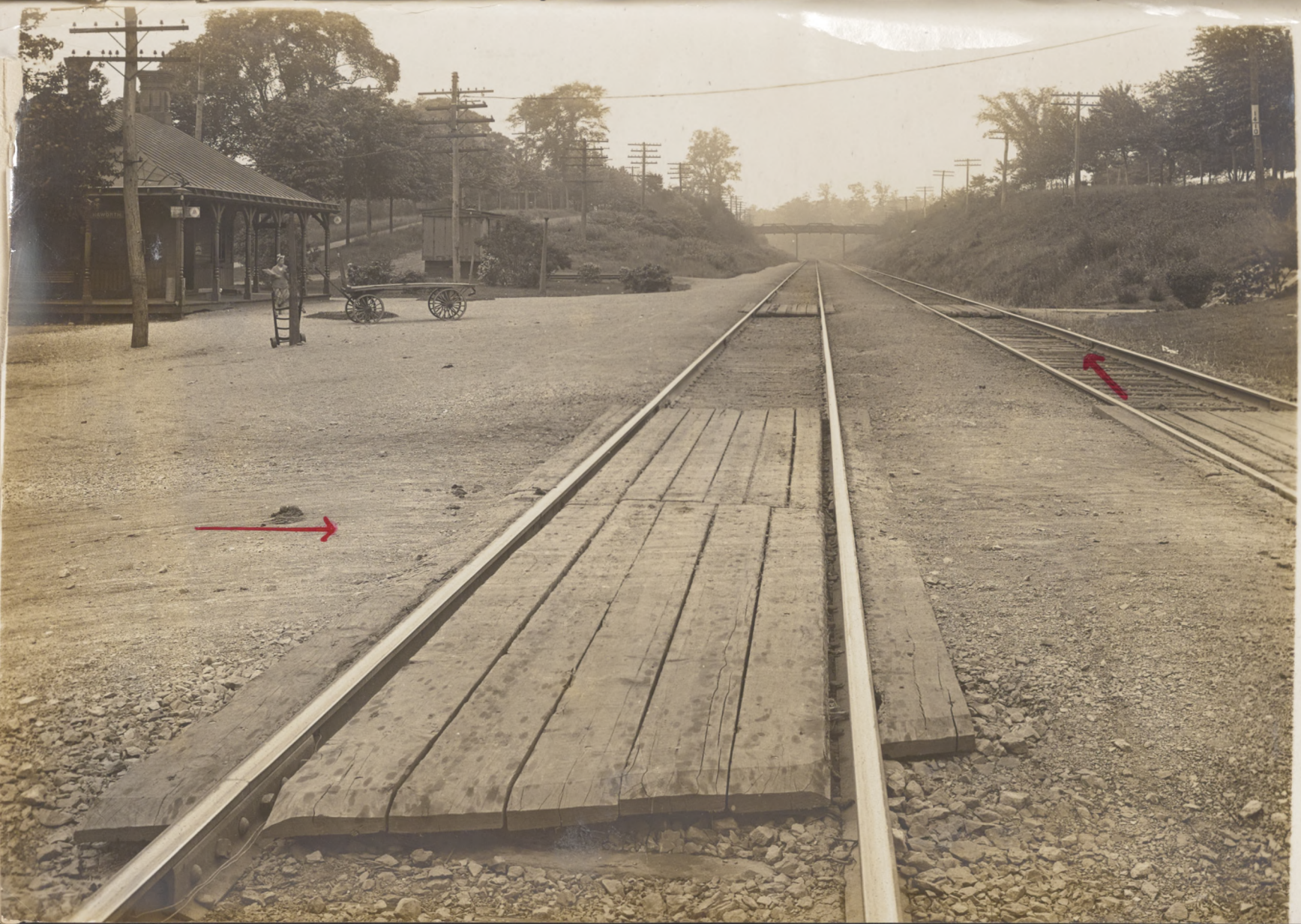
Haworth N J 4-15-15. Case M Cattf Plate No 4503 Detail view of crossing planks over North bound track looking South.
