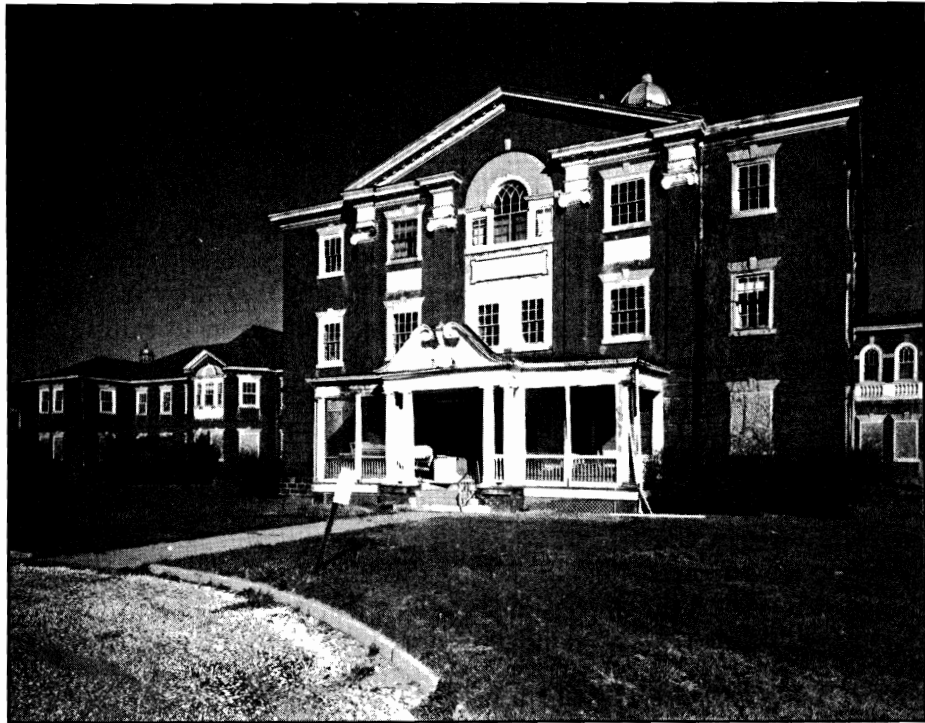
Figure 12 Cumberland County Hospital (1899), a massive Georgian Revival building composition, is one the most formal in the area and currently unused.
