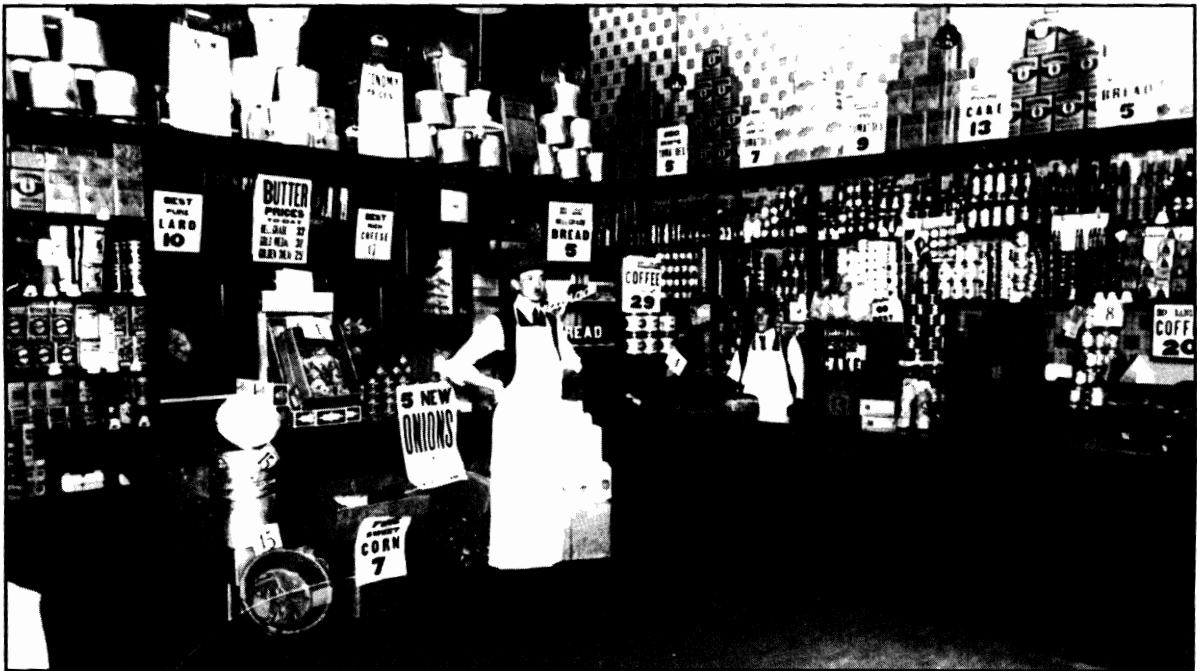
Figure 80. During the 19th century almost every town in South Jersey had general stores such as this one in Millville. Wettstein , late 19th century.
