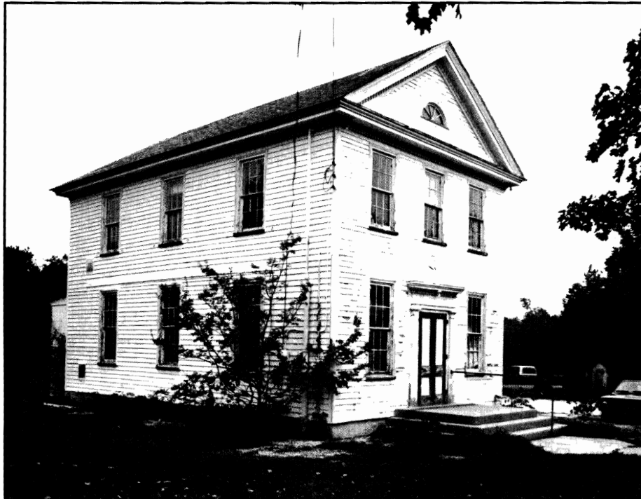
Figure 102. Mauricetown Academy (1860). The entry is in the gable end, secondary doors to the side; the pediment has a dentiled cornice and semi-lune.
