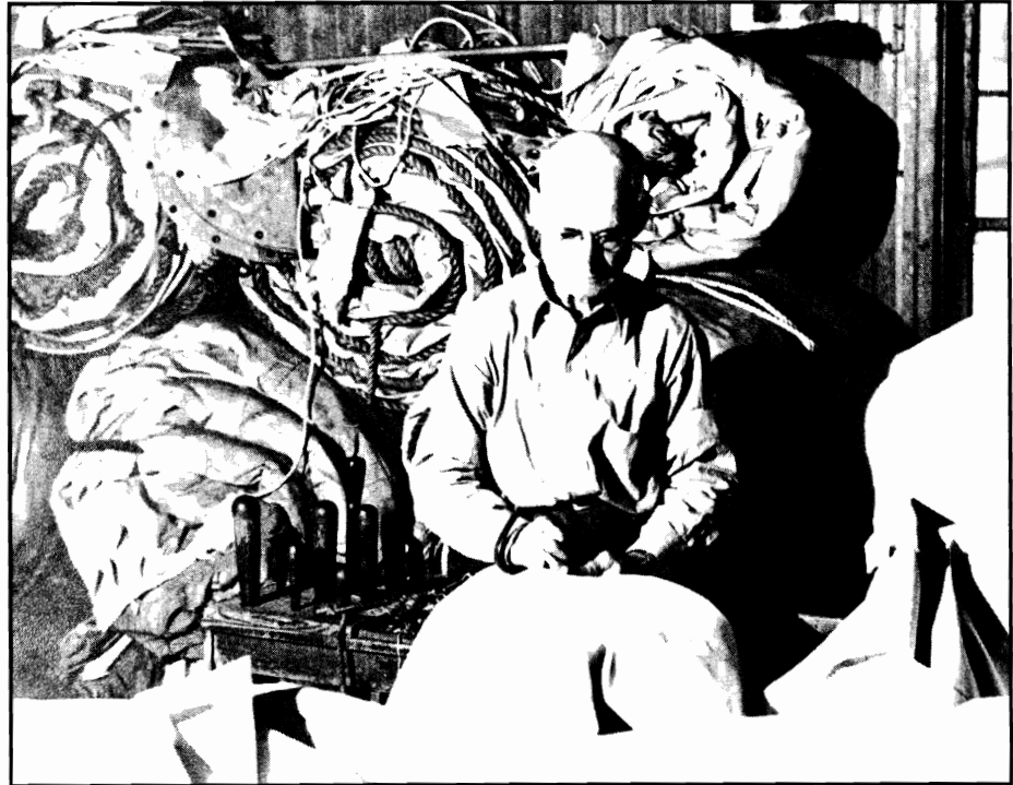
Figure 28. Sailmaker Ed Cobb working in the sail loft of a building that is extant in Bivalve. Rutgers Collection, early 20th century.
