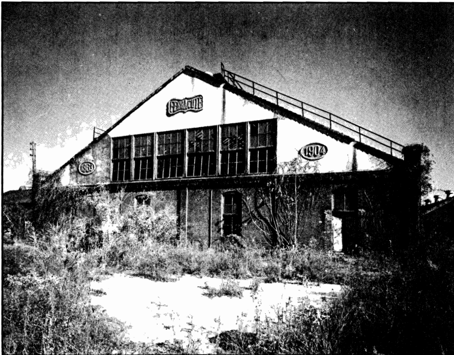
Figure 70. This largest of the Ferracute buildings is structurally sound, but the presses and other equipment have been removed.
