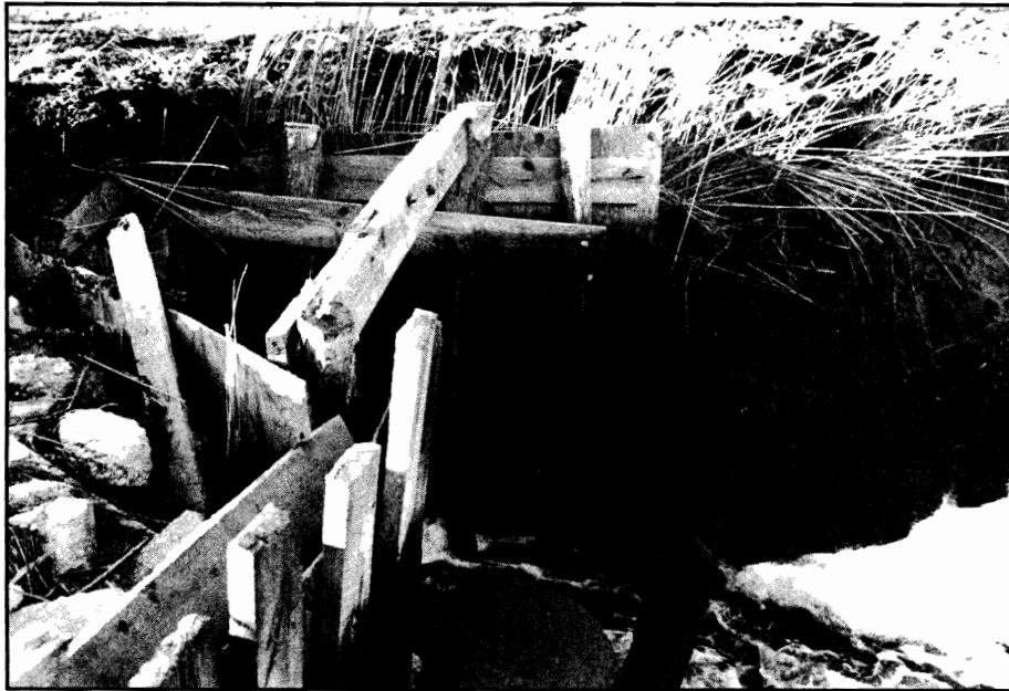
Figure 54. Sluice gates around a drain pipe let water escape from fields at low tide; as the tide rises, the gates press shut so as not to flood the fields. Sebald.
