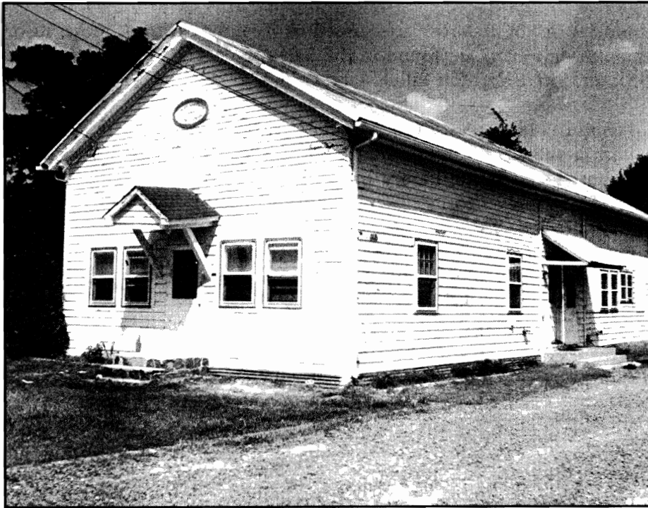
Figure 105. Lower Hopewell School (1859) has been somewhat altered, but it retains the vernacular Greek Revival form popular during the 19th century. Leach.
