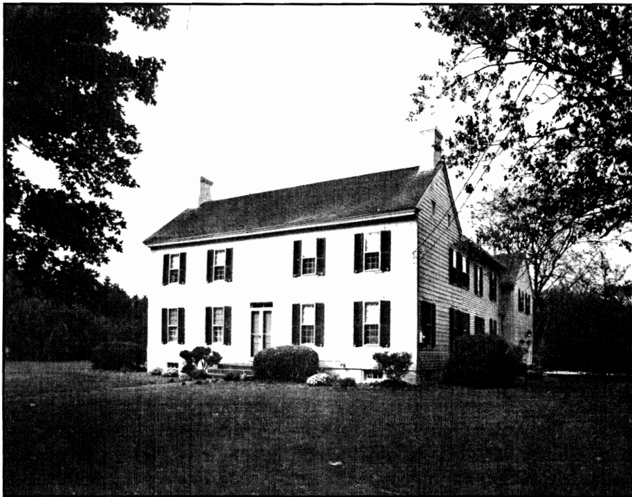
Figure 45. Christopher Ludlam House (1776), though plain, is an ordered, Georgian five-bay block with gable-end chimneys, center door, and rear additions.
