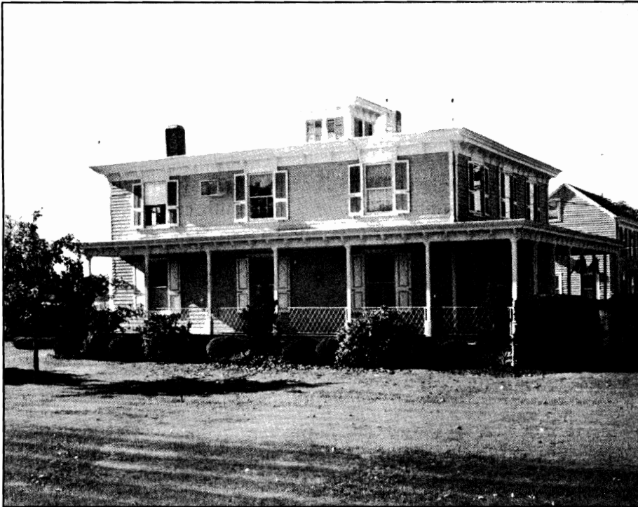
Figure 16. Padgett Funeral Home (19th century) is characterized by its boxy lines, flat roof and Italianate detailing.
