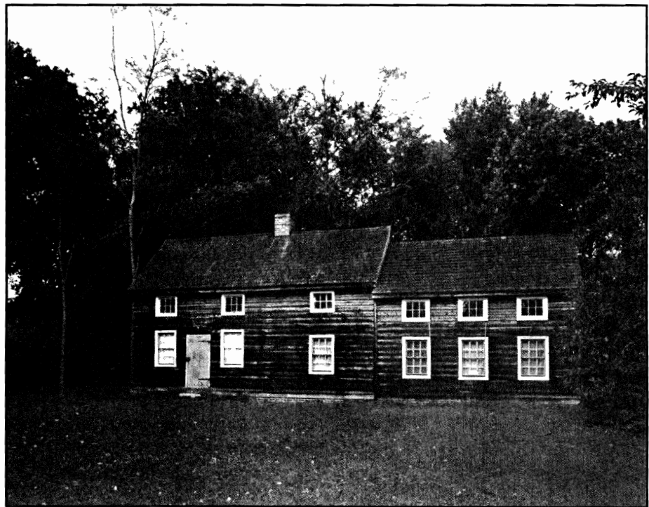
Figure 44. Thomas Ludlam House (1743), originally a hall-and-parlor plan, has been enlarged with the addition of four bays and relocated below Dennisville.
