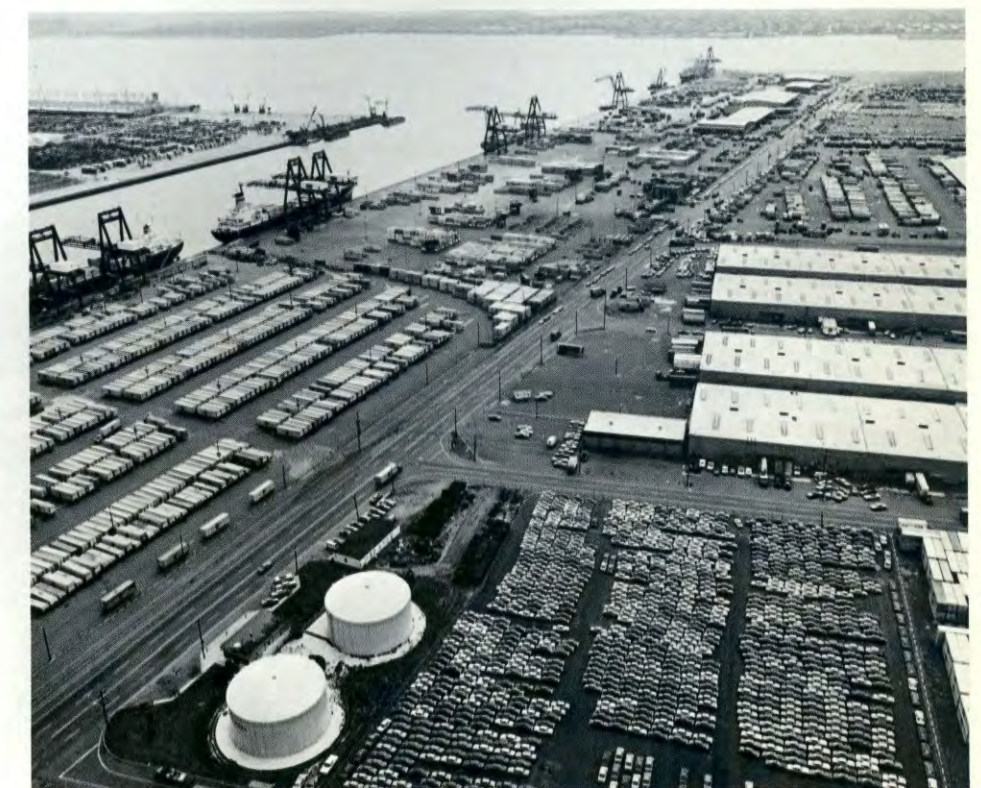
Elizabeth Marine Terminal, Container Capital of America, provides hundreds of acres of upland area for handling and storage of cargo.
