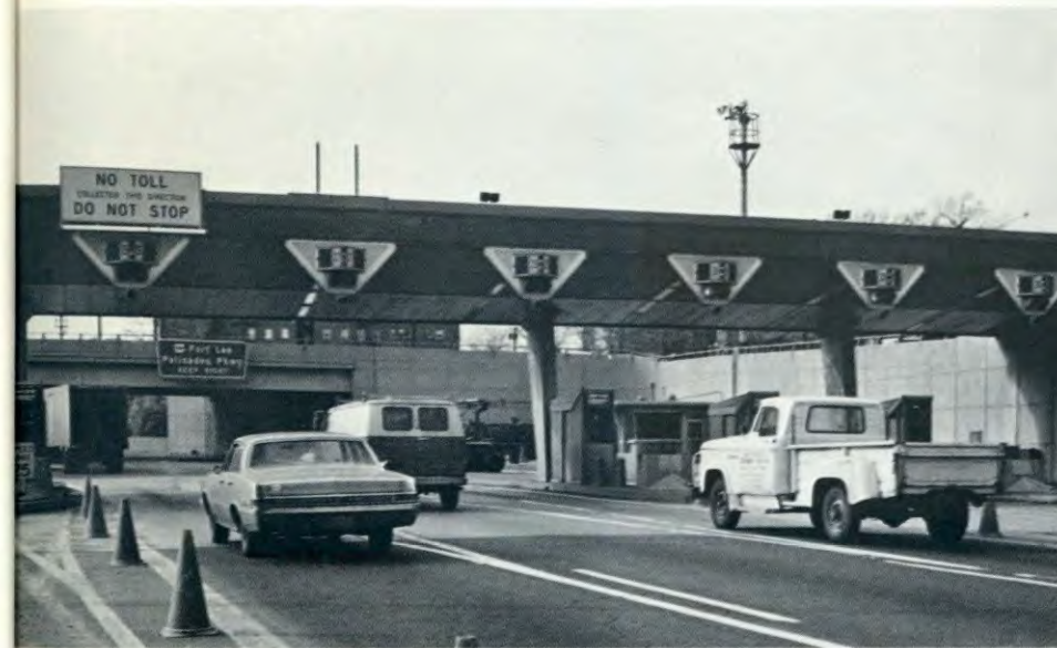
The introduction of one-way tolls at Port Authority crossings and other Hudson River crossings eased congestion and expedited the flow of traffic.
