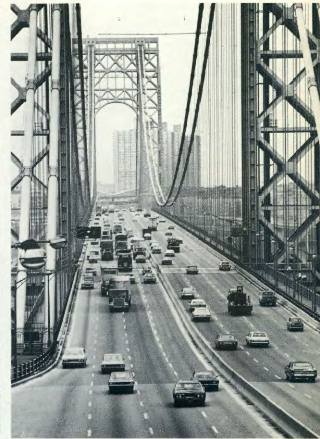
Concrete and steel median barrier was installed on upper level of George Washington Bridge in 1970.
