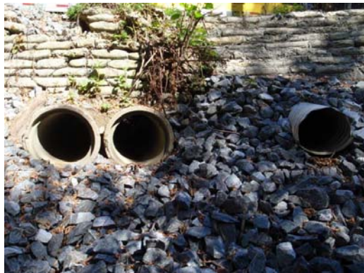
Figure 3. Clay pipe culvert: view of outlet side
