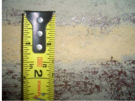
Figure 6. Repair of a small gap caused by pipe settlement
