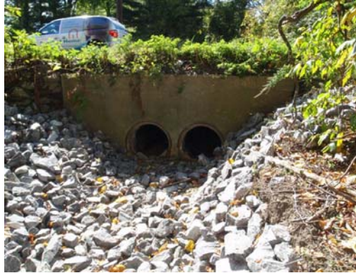
Figure 2. Clay pipe culvert: view of inlet side
