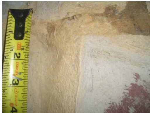
Figure 8. Repair of a cracked corner gap caused by pipe settlement
