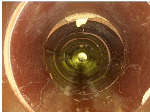
Figure 4. Clay pipe culvert: view of interior
