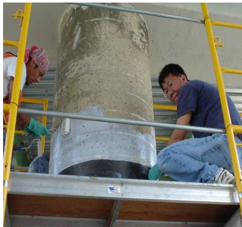
Figure 1. Carbon fiber wrapping of column with inorganic polymer
