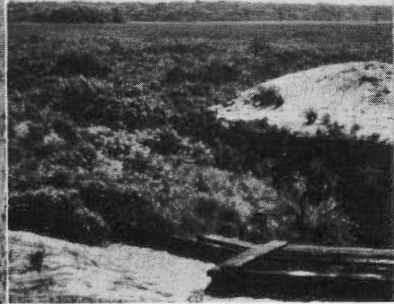
Then, dikes constructed to control
