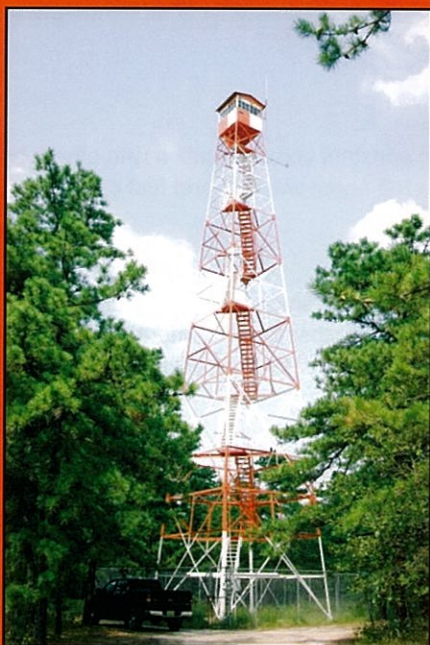
Cedar Bridge Tower, Ocean County
