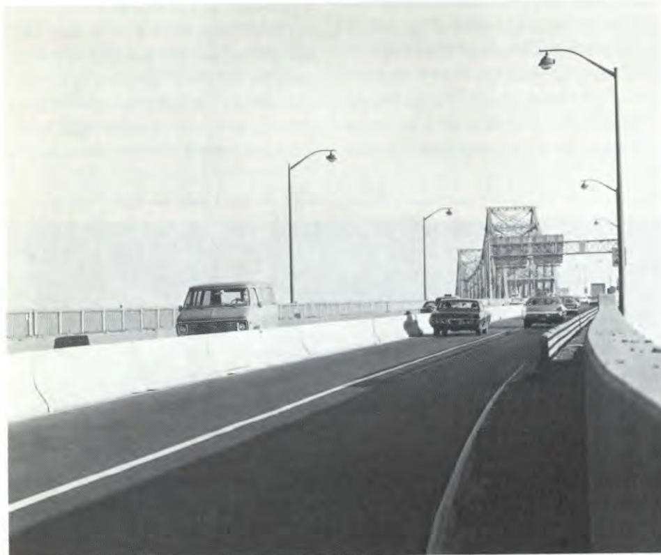
Concrete and steel median barrier was installed on the Goethals Bridge and its approach roadways in 1972.
