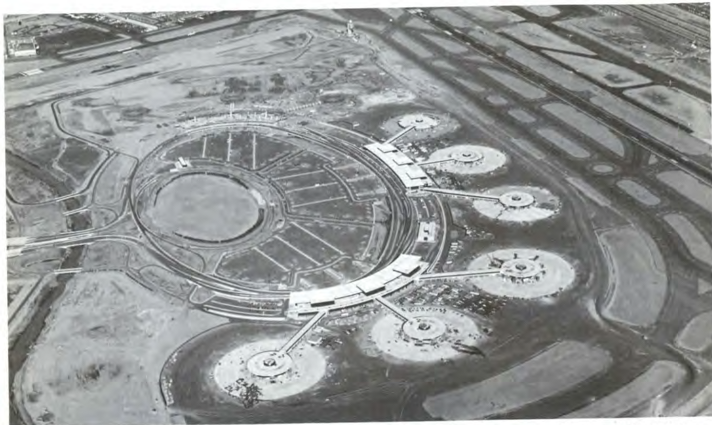
Structural work on Terminals A and B of Newark Airport Redevelopment Program was completed along with parking lots, roadways and lighting systems.
