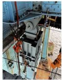
Left to right: 3D models of the telescope temporary rocker links and a photo of one installed on the bridge (Skanska USA Civil)
