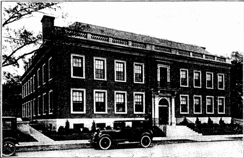
The Metcalf Memorial Building at Orange containing Offices of the Welfare Federation, eight of the Federation Agencies, the Council of Social Agencies, and the Dental Clinic
