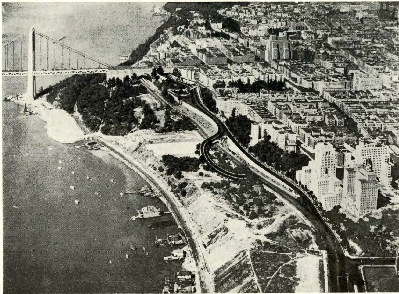
Hudson River Bridge. Perspective of New York Approach and Connections to Riverside Drive
