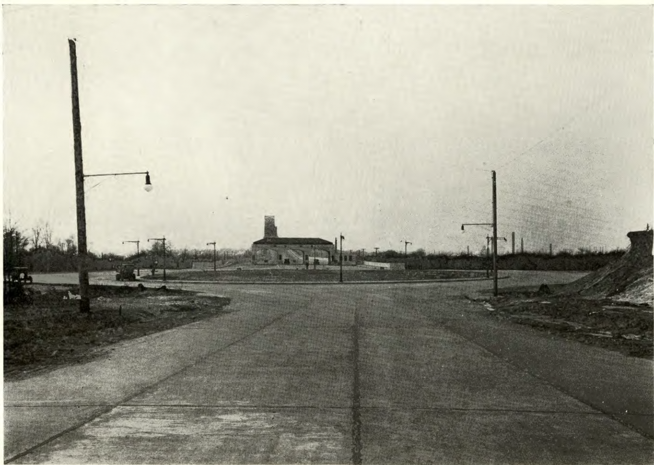
Outerbridge Crossing. Tottenville Plaza, looking west toward toll booths and bridge
