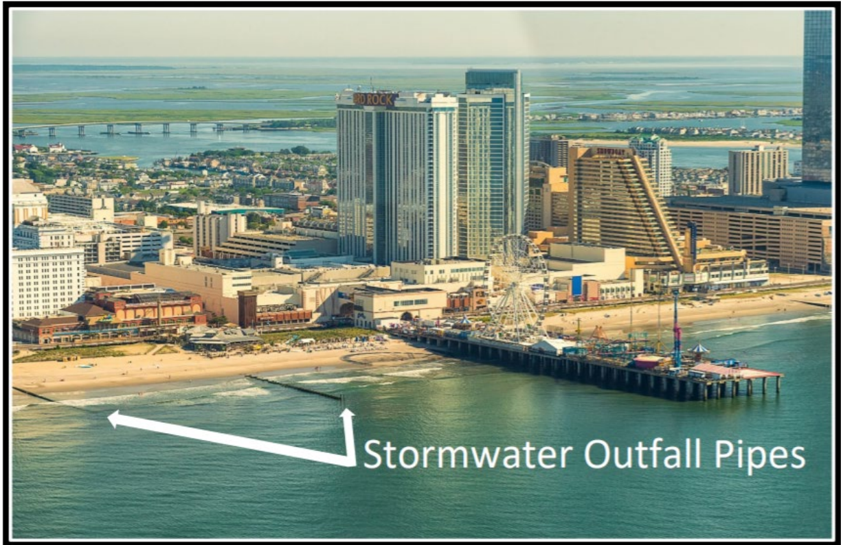
Figure 10: Stormwater Outfall Pipes in Atlantic City, Atlantic County
