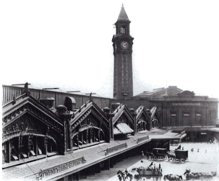
Hoboken Ferry Terminal (date unknown)
