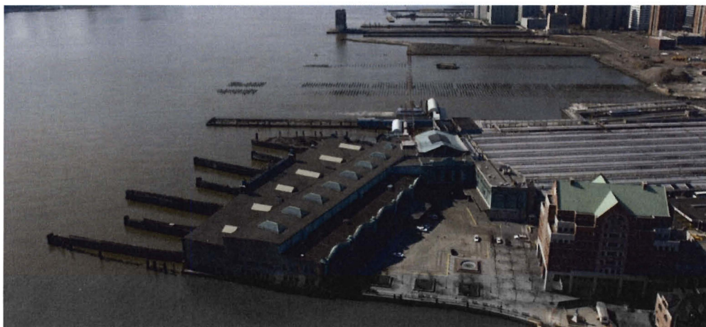
Hoboken Terminal, Aerial View from North, 2004
