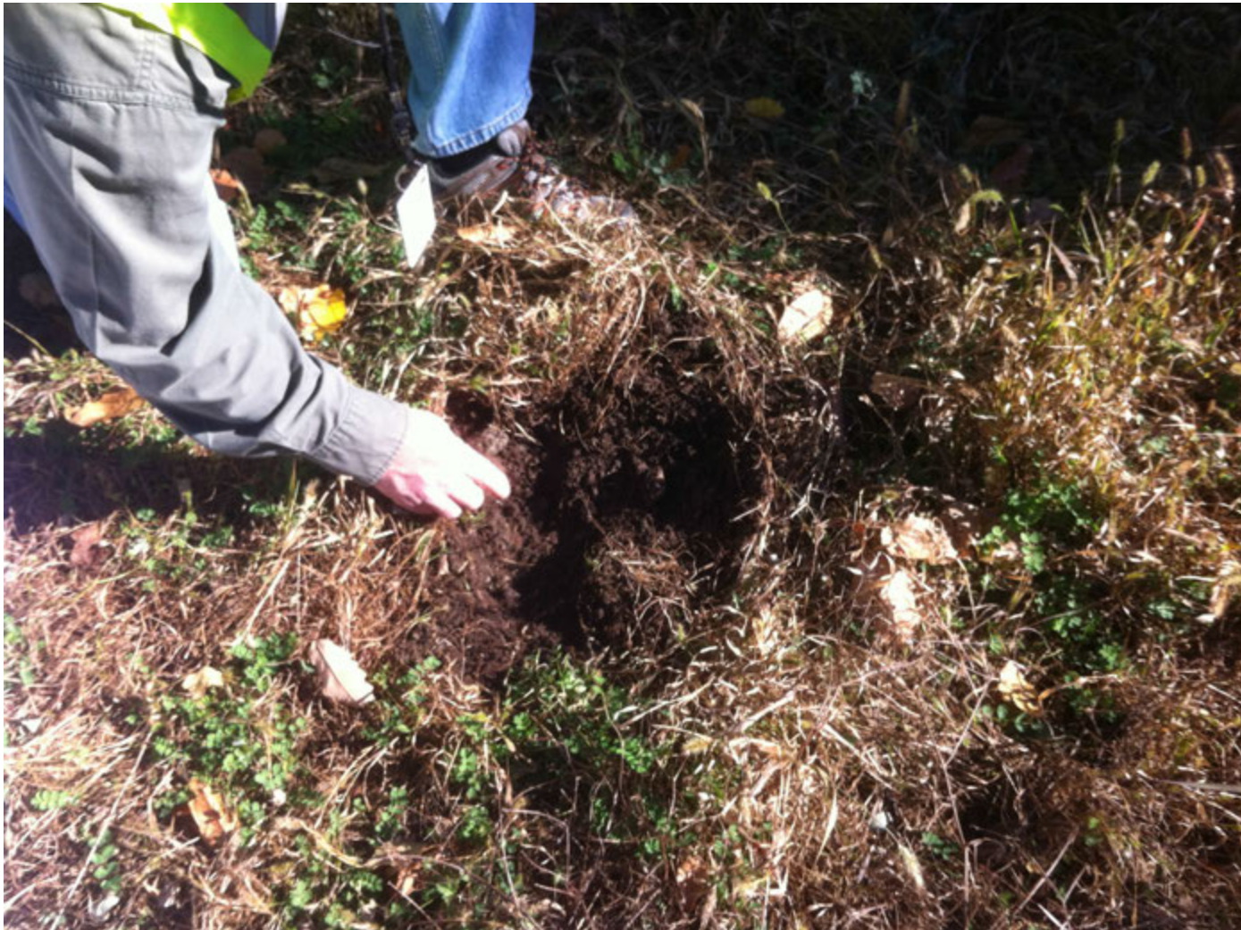
Ground and soil detail of "shot rock" area.
