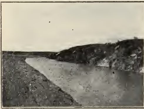
Canadian Pacific Railway Company's irrigation project, Calgary, Canada.
