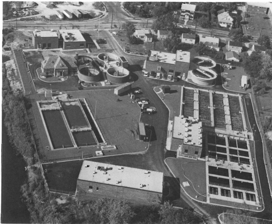
Construction of wastewater treatment facilities is one program which will benefit from the New Jersey Infrastructure Bank.
