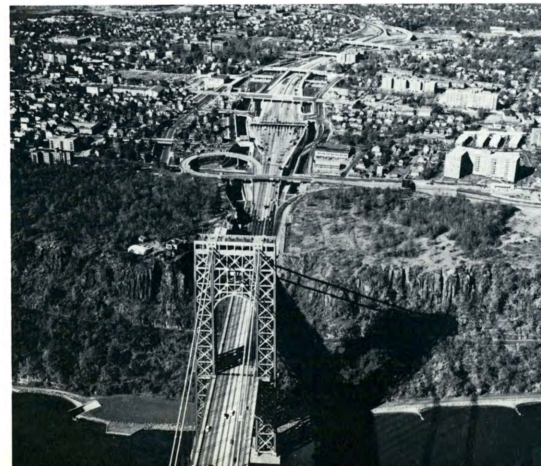
The New Jersey approach system provides direct connections to and from the George Washington Bridge and Highways US-1, US-9, US-9W, US-46, NJ-4, the Palisades Interstate Parkway, and the Bergen Expressway (scheduled to open in 1964). The portals of two, three-lane lower level approach tunnels can be seen in the broad plaza area, and beyond them, the new bridges which carry local north and south-bound traffic over the main approach roadways.
