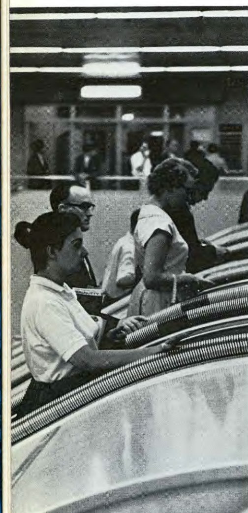
The escalators shown here have been supplemented by the installation of 29 high-speed motorstairs for the conveyance of patrons to and from passenger levels.
