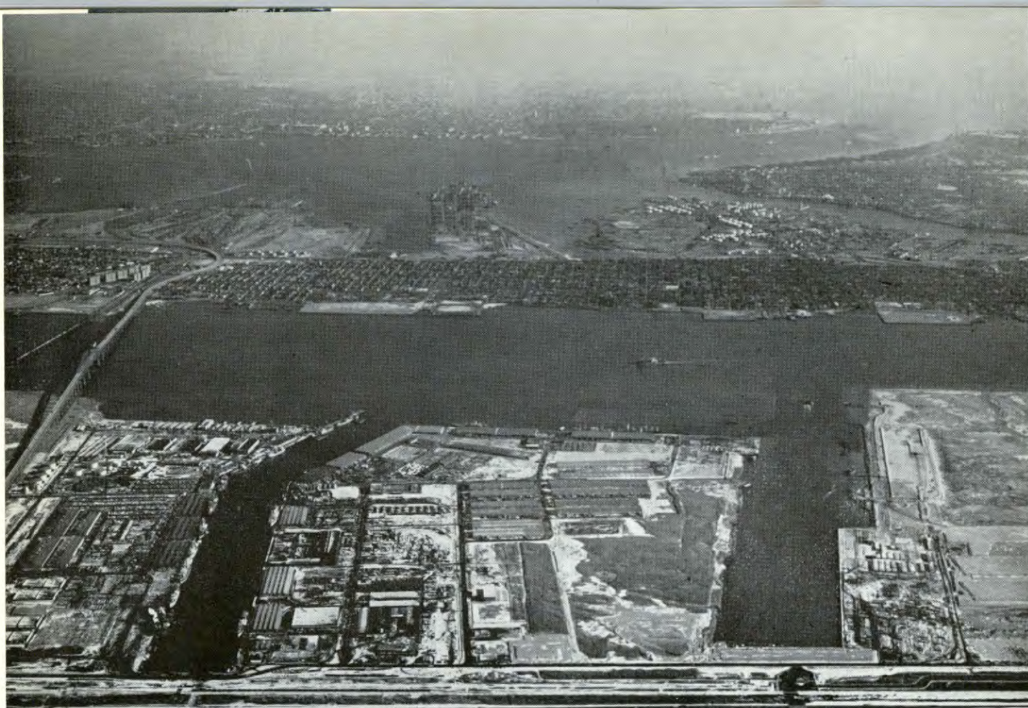
Port Newark, still the busiest of the Port Authority's marine terminals, and the Elizabeth-Port Authority Piers are shown as they appeared in December, 1962. Several months earlier, the Elizabeth-Port Authority Piers had dedicated the opening of the first stage of its $150,000,000 development project. The Master Plan for the Elizabeth facility calls for the ultimate construction of 24 deep-sea berths.
