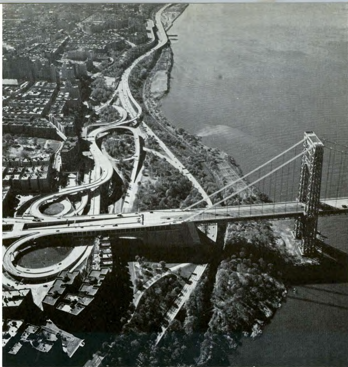
On the New York side of the George Washington Bridge a system of north and south loop ramps provides motorists with wider and more direct connections to both levels of the bridge and to major highways leading to destinations north, south and east of the expanded structure. To the left of the anchorage can be seen the beginning of the 12-lane, depressed George Washington Bridge Expressway which leads to the new George Washington Bridge Bus Station, the Harlem River Drive, Amsterdam Avenue, and the Cross Bronx Expressway.
