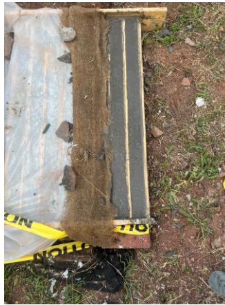
Figure 19. RS samples curing with burlap
