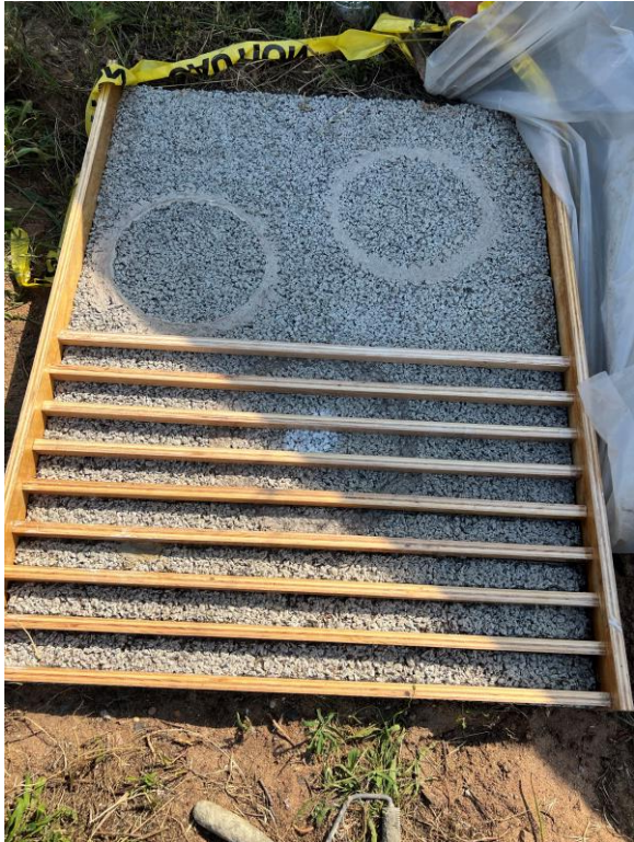
Figure 15. Formwork for porous slab
