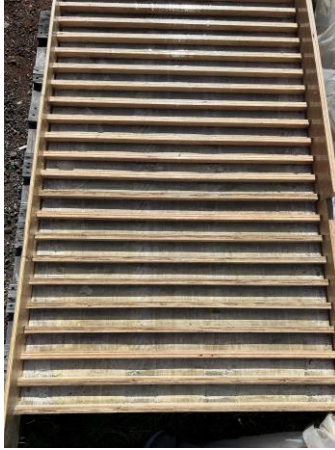
Figure 16. Formwork for Plain Slab
