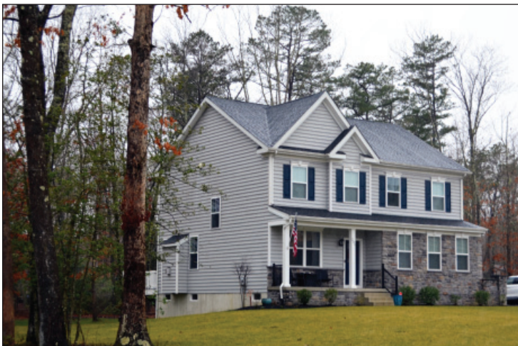
Above: The housing development above was built with an alternate design wastewater treatment system in the Pinelands Area of Tabernacle Township. Photo/Paul Leakan
