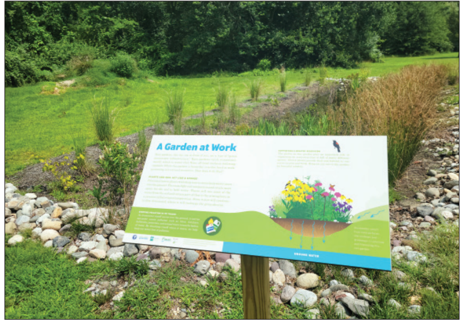
Above: This rain garden that was installed at the Hammonton Lake Park is an example of a green infrastructure measure that will be required for minor development under the Commission's new rules. Photo/Paul Leakan
