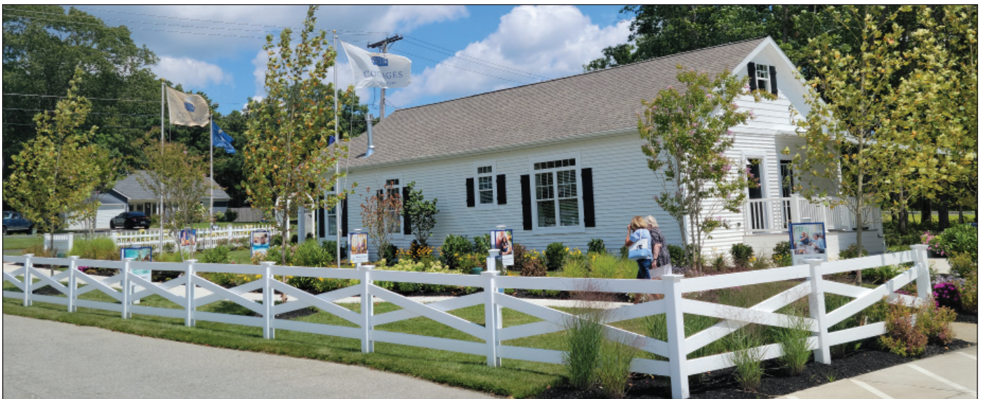
Above: Prospective buyers can tour a model cottage at The Cottages at Compass Point, a development that will include 212 single-family detached homes and a 13,500-square-foot clubhouse in Barnegat Township’s Regional Growth Area and required the use of 16 Pinelands Development Credits (or 64 rights).
