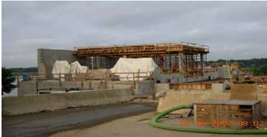
PRIMARY TREATMENT BUILDING UNDER CONSTRUCTION Photo Courtesy of Milford-Housatonic WPCF
