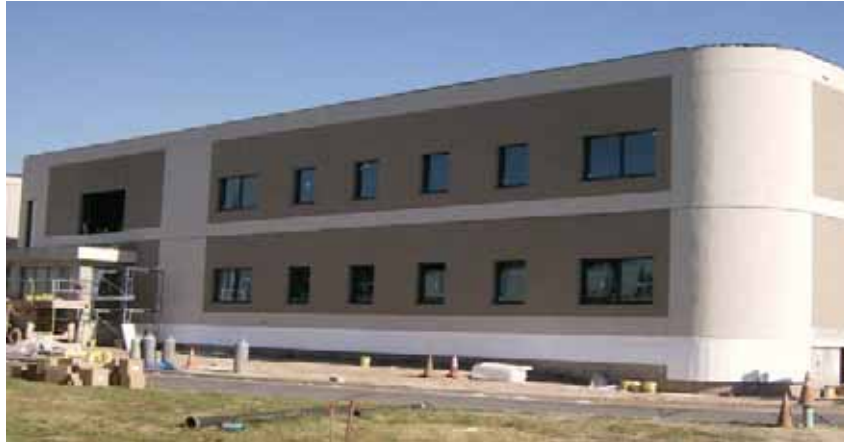
NEW LABORATORY AND OFFICE BUILDING Photo Courtesy of Joint Meeting
