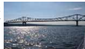
TAPPAN ZEE BRIDGE Photo by G. Spencer
