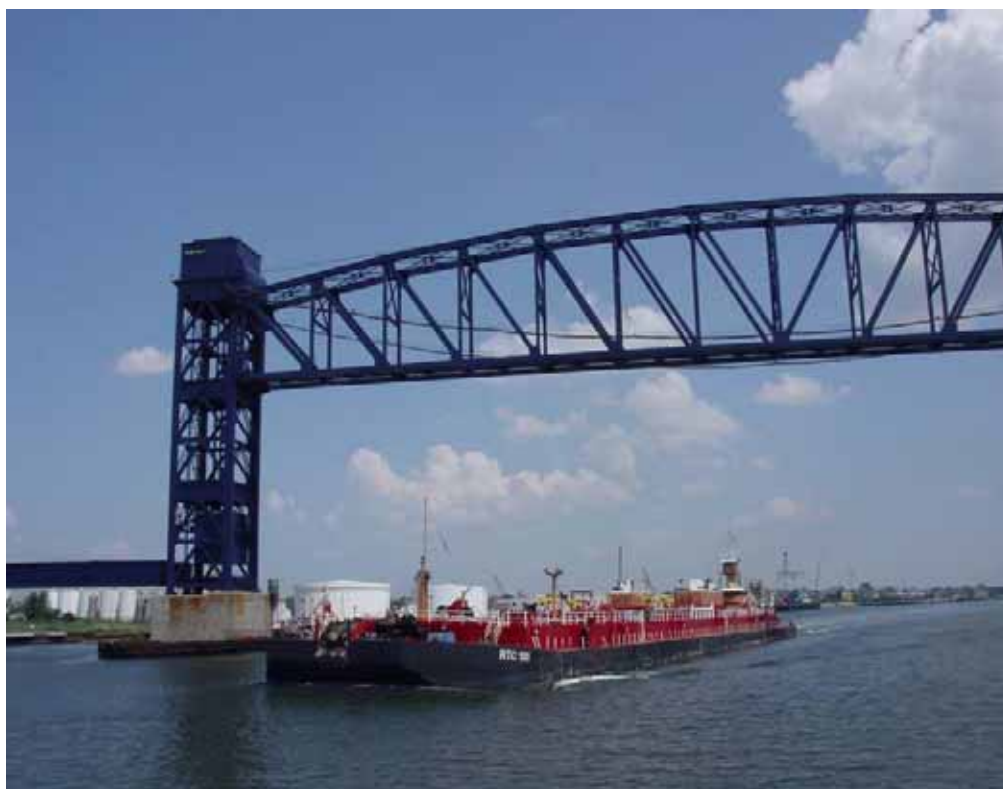
ARTHUR KILL LIFT BRIDGE, AUGUST 2007
