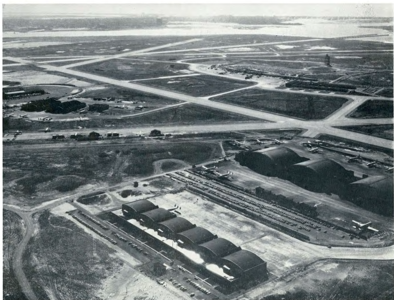
Major development activity is taking place at New York International Airport where the accent is heavy on construction. Recently completed Hangar 6 is in the foreground and the superstructure of Hangar 7 is at the extreme upper left. Work on Hangar 8, first of a number of hangar developments in the Airport's central operating area, was begun in September. Negotiations for three other hangars were concluded during 1953.
