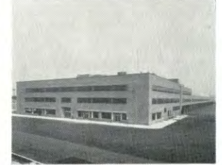
NEWARK UNION MOTOR TRUCK TERMINAL
