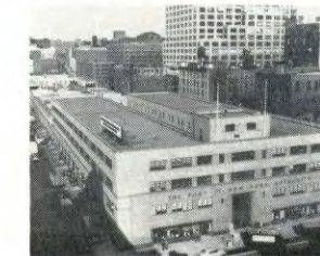
NEW YORK UNION MOTOR TRUCK TERMINAL
