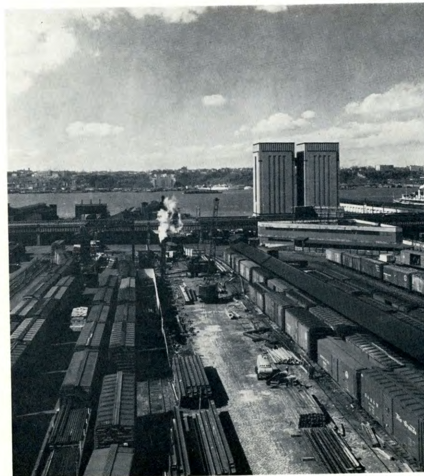
Construction of the land shaft at the New York end of the Third Tube project was started in February, 1953 — when this picture was taken — in Thirty-eighth Street just east of Twelfth Avenue following ground-breaking ceremonies in 1952. Excavation for the New Jersey shaft was begun in June, 1953. The line of the new tube will run from 130 to 190 feet south of the present two Lincoln Tunnel tubes whose position is marked by the towering ventilation buildings to be seen here on either bank of the interstate Hudson River. The Third Tube will be driven beneath the Hudson by the shield method which was used in building the Holland Tunnel and the existing tubes of the Lincoln Tunnel. The under-river phase of the work will begin on the New Jersey shore in April, 1954 when the shield will be assembled in the New Jersey shaft under Kings Bluff.
