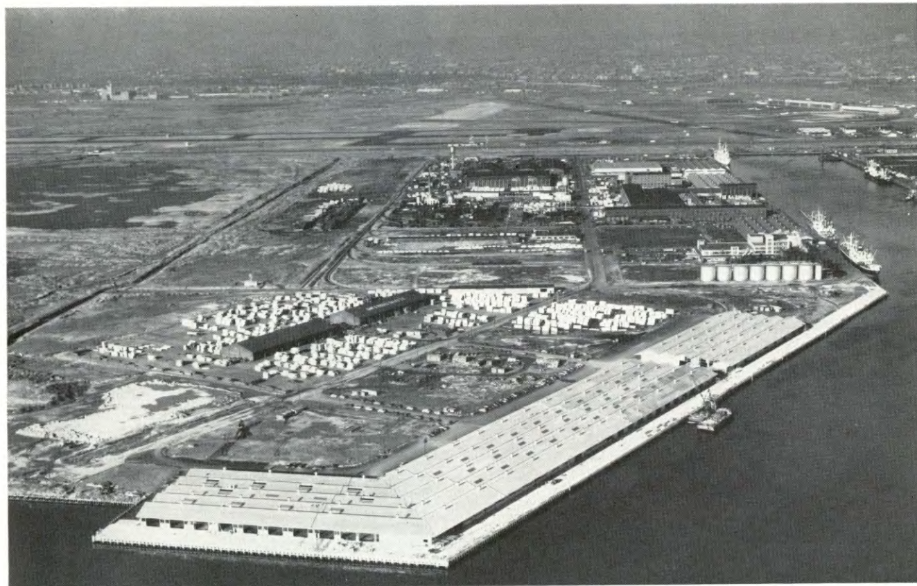
When the $6,000,000 marine terminal we are building for the Waterman Steamship Corporation at Port Newark is completed, common carrier foreign service to North Europe and the Far East will be available here for the first time. The new terminal, shown in this view, is expected to be completed and opened for operation by April, 1954.
