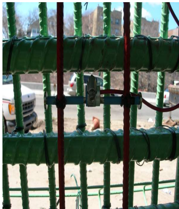
Figure 27. Close-up View of the Sensors in Drilled Shaft #3
