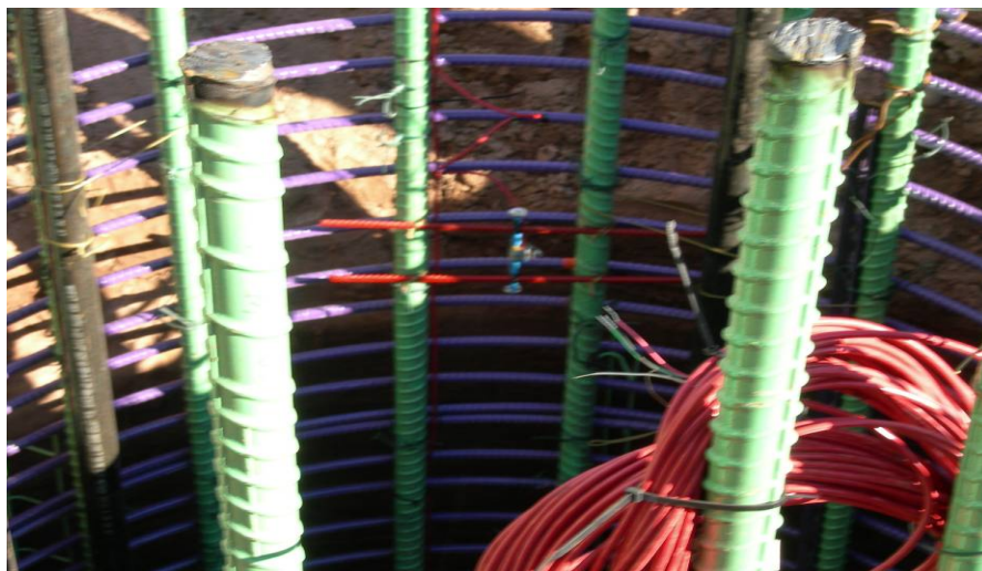
Figure 20. Model 4200 Gage After Cage Placement
