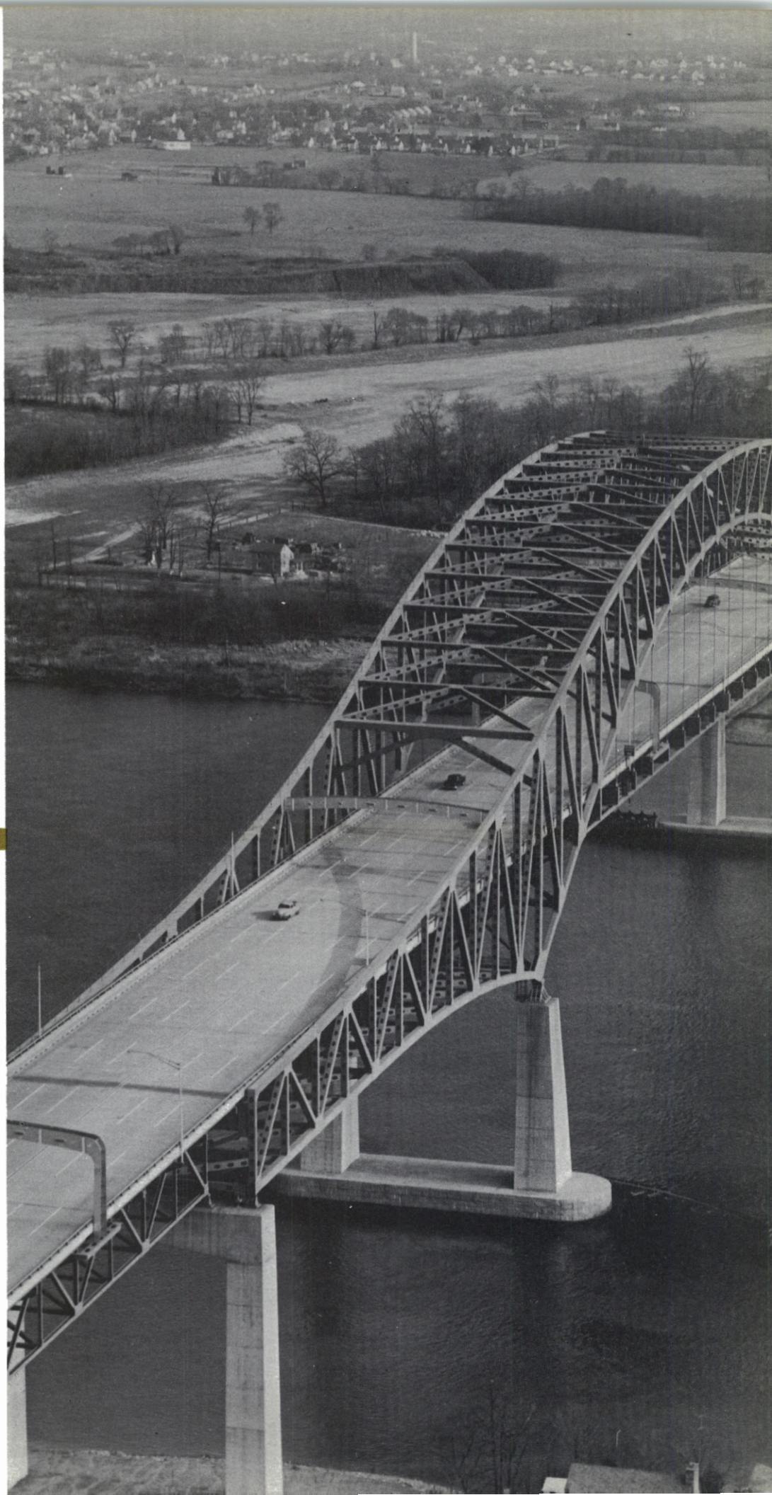
New Delaware River Turnpike Bridge connecting New Jersey and Pennsylvania Turnpikes
