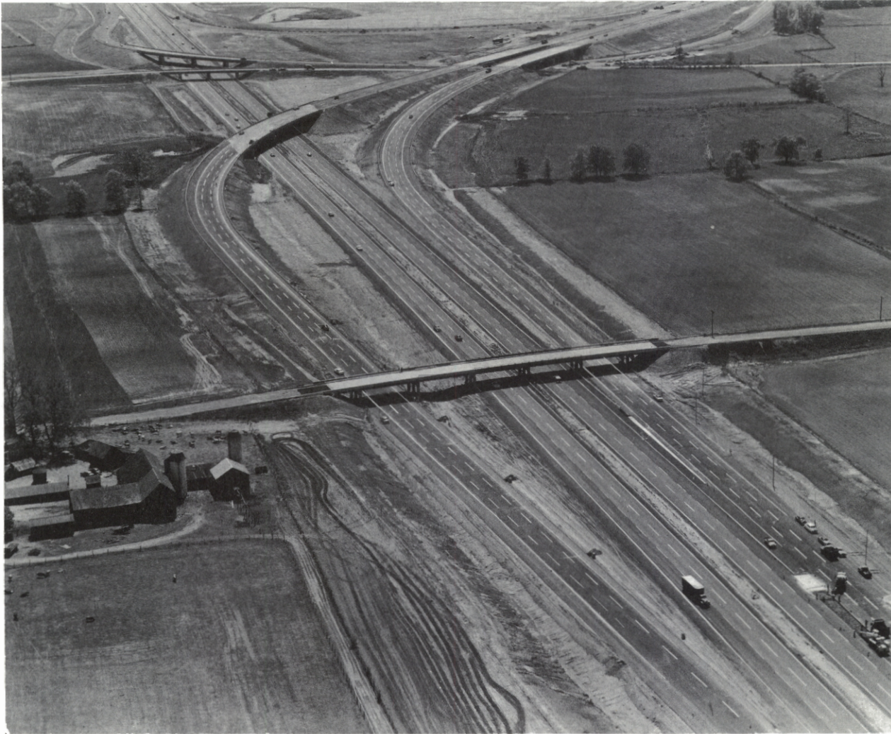
Southbound on Turnpike where direct connection is made to Pennsylvania extension
