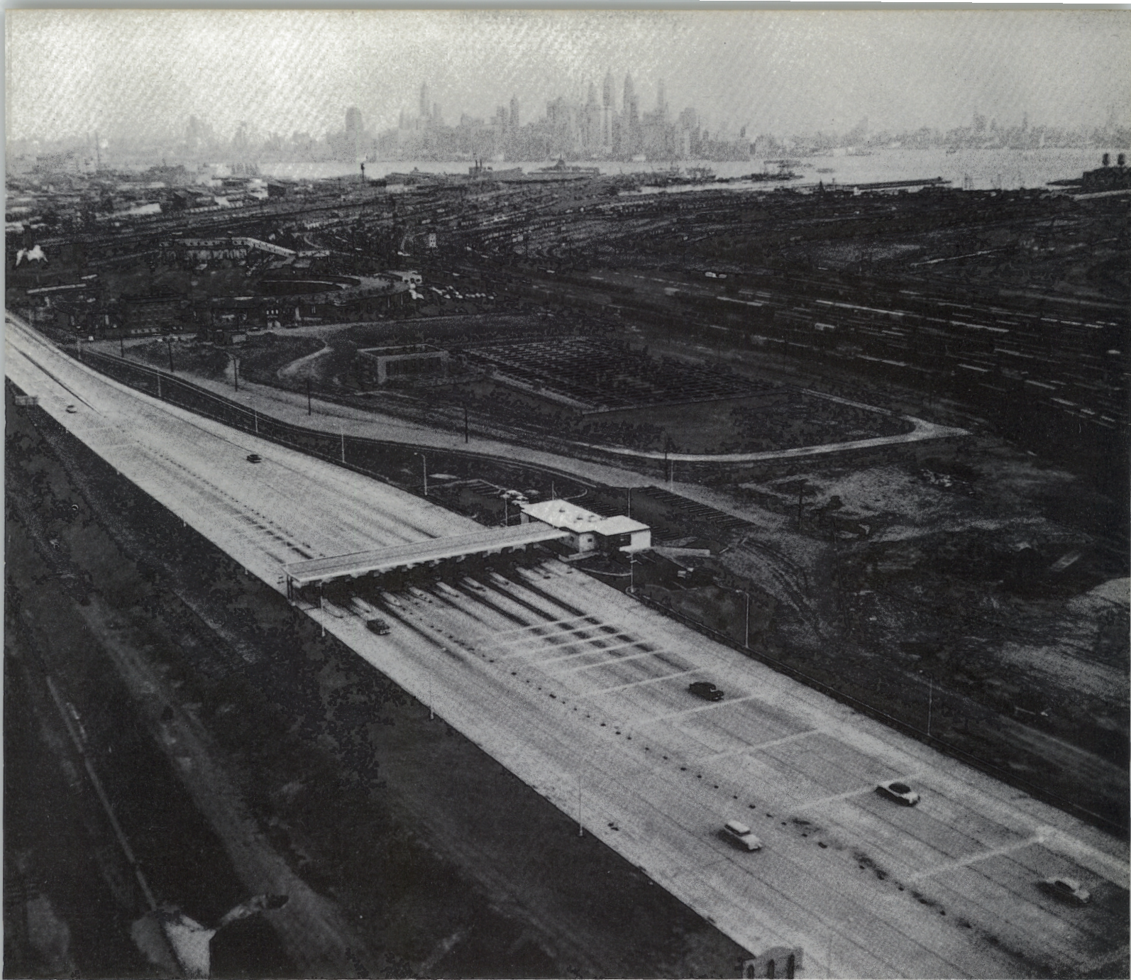
Holland Tunnel interchange of Newark Bay-Hudson County extension. Downtown New York City in background
