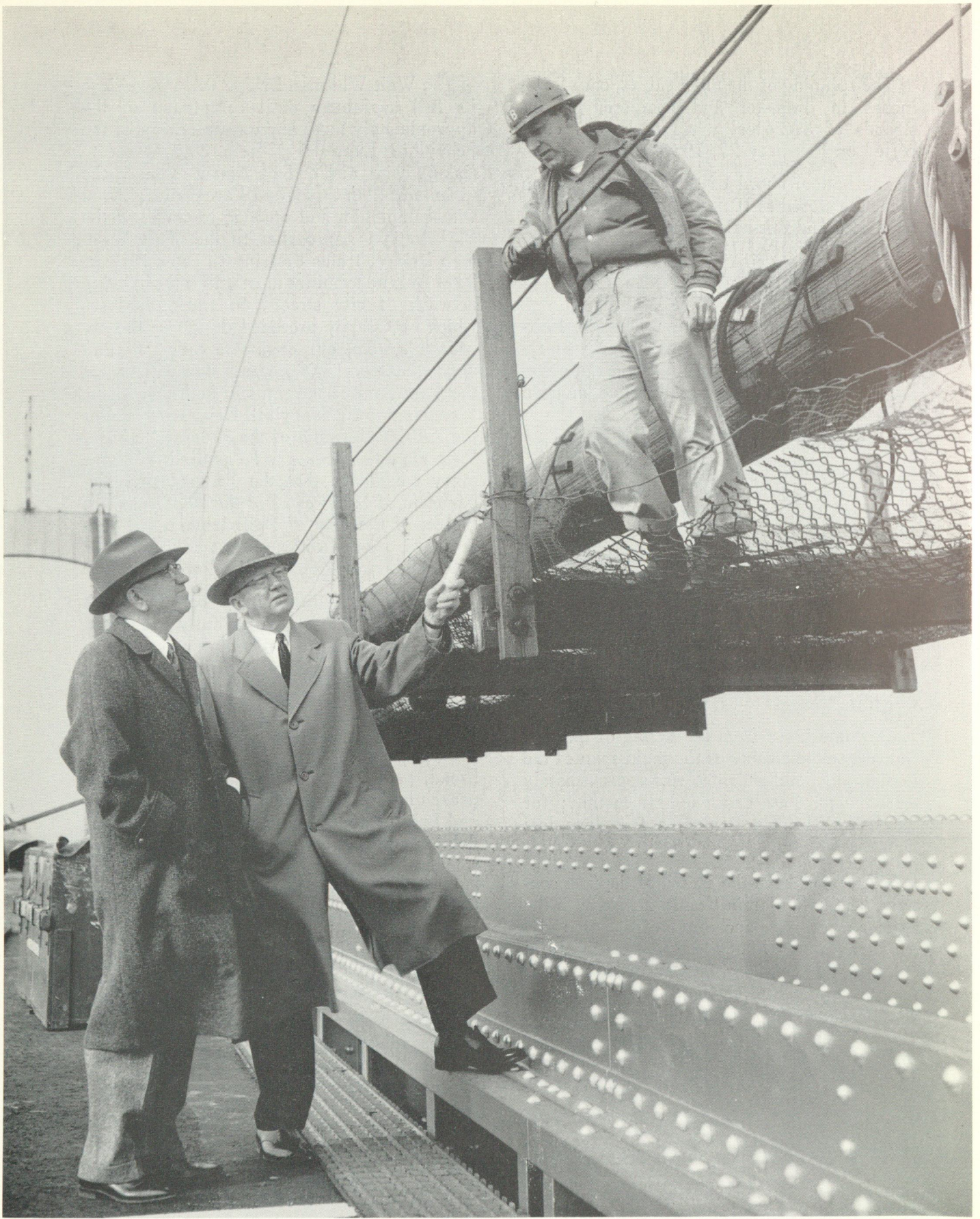
FIRST OFFICIAL CROSSING OF WALT WHITMAN BRIDGE, NOVEMBER 21, 1956 Port Authority Chairman, Weldon B. Heyburn, and Vice Chairman J. William Markeim chat with workman 12
