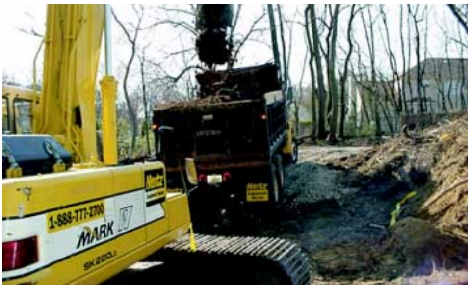
The contaminated soil is placed in trucks for off-site disposal.
