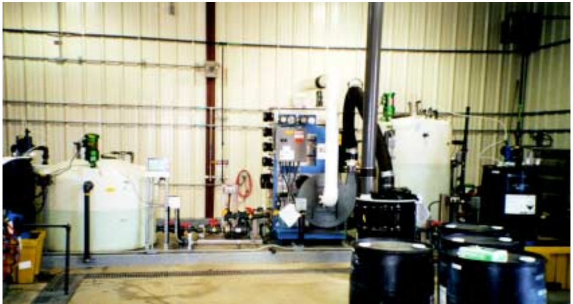
A view of the inside of the Ellis Property ground water treatment plant, showing from left to right the acid treatment tank, air stripper and effluent storage tank.
