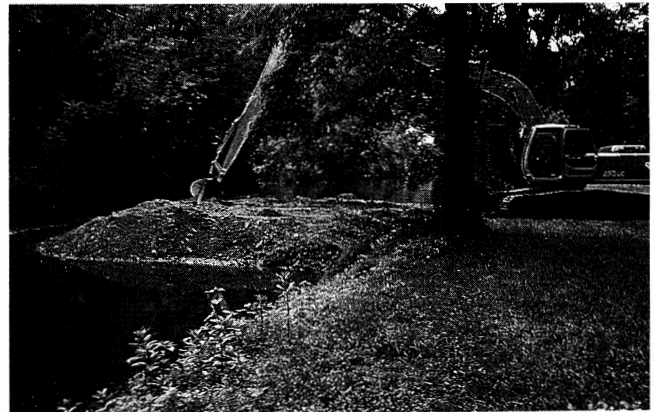
The Waterways and Embankments unit removed over 2700 cubic yards of material from the Brookville Creek Inlet in Delaware Township, Hunterdon County.
