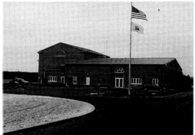
The Manasquan Administration building houses a reservoir pumping station and the maintenance and administrative offices for the system in Wall Township.
