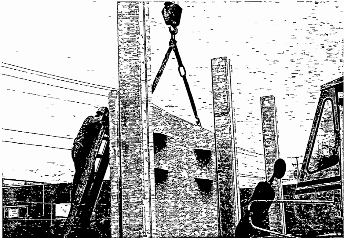
Fig 16 Panel Fig 15 being bolted from the residential side with the bush hammer side to the post
