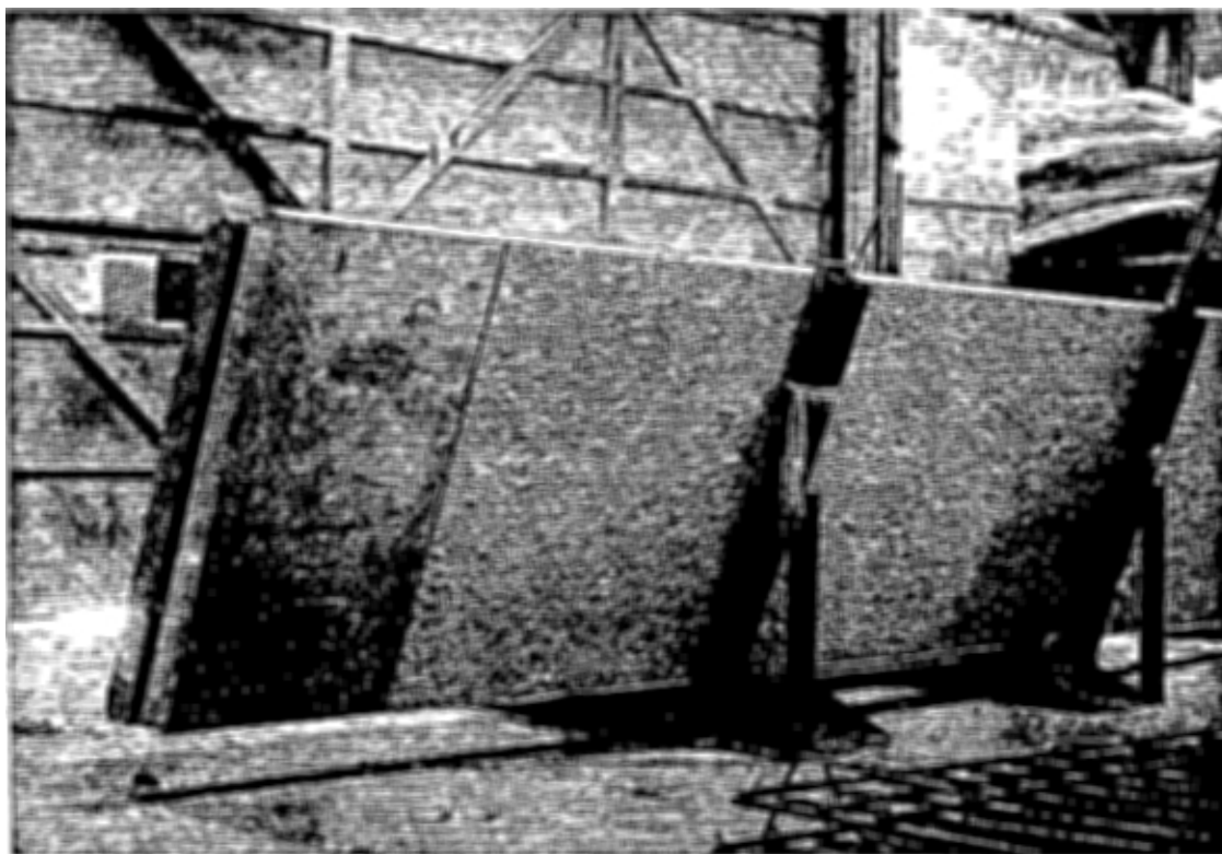
Fig 2 Bush hammer (highway side) 4 ft. panel with smooth end treatments which rest against the posts
