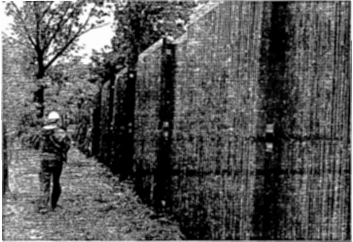
Fig 46 View of highway side wall
