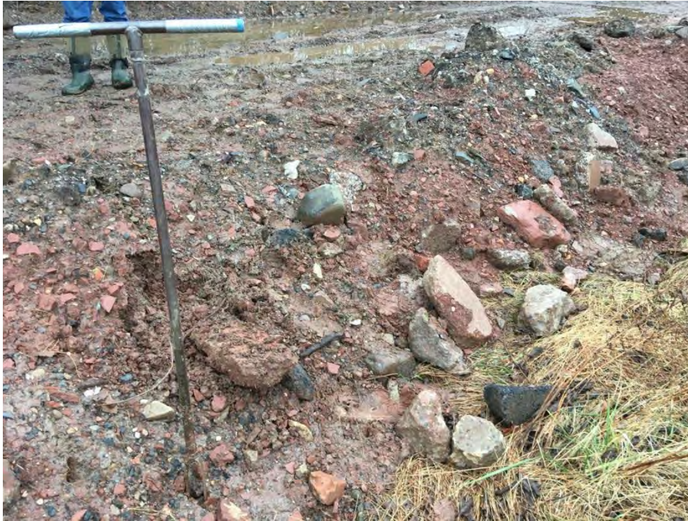
Photo 7. HTM on western edge of farm lane; some ponding is visible.
