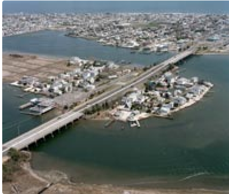
This aerial view is of the existing trestle bridges over West and East Thorofares.
