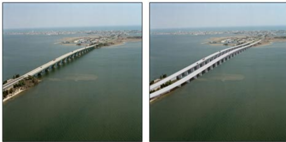
The existing Manahawkin Bay Bridge is on the left and the proposed twin bridges are on the right.
