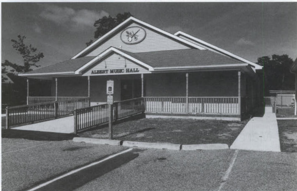
The new Albert Music Hall, located in Waretown, opened its doors on January 5, 1997, four and a half years after fire destroyed the original building. The 6,000-square-foot music hall, which is air conditioned, smoke- and alcohol free and handicapped accessible, seats 350 people.
