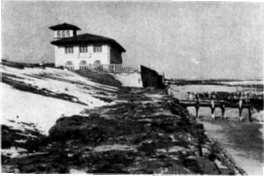
Same View—After Installation of Coast Protection Structure
