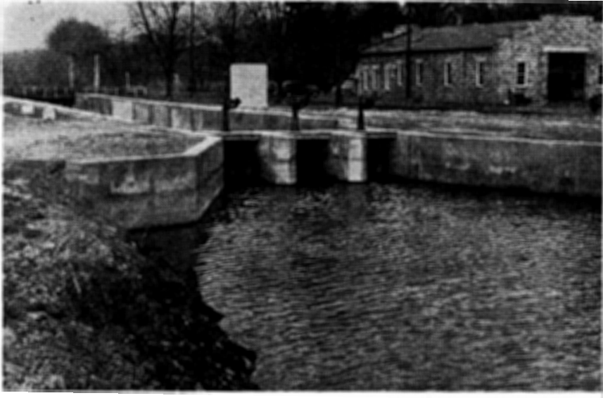
D. & R. Canal—Kingston—Lock and Control Gates after Reconstruction
