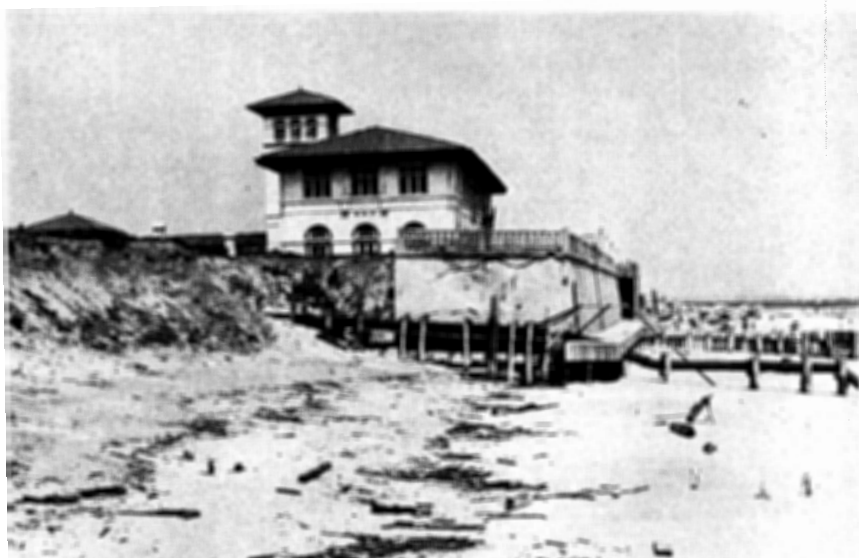
Beach—Vicinity of Deal Casino—Before Installation of Coast Protection Structure
