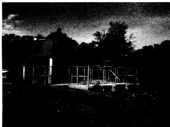
The Ten Mile Pump Station located in Franklin Township, Somerset County, was brought back to operational status after a lightning strike damaged the electrical service.
