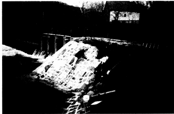
Extensive rehabilitation of two culverts and adjacent walls was undertaken at Prallsville in Hunterdon County
