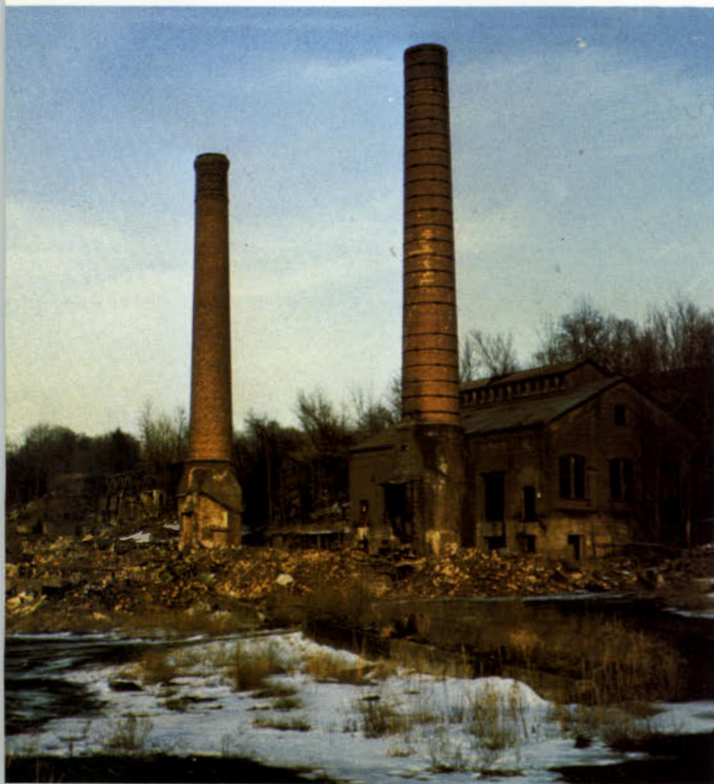
Reduced to rubble and sold for scrap, these are the only remains of a zinc mine and mill that produced a half-billion dollars' worth of ore in 125 years of operation.
