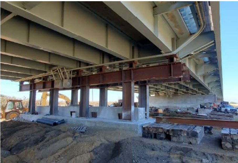
Temporary steel supports installed. The supports raised the bridge 1/8" to allow removal and installing of a new concrete pier.
