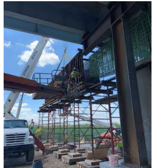
Crews construct concrete forms in preparation of pouring the new concrete pier.
