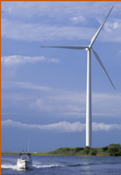
Wind Turbine, Atlantic City, NJ
