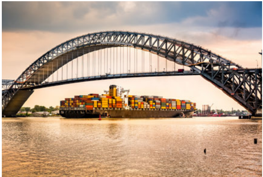
Bayonne Bridge, NJ
