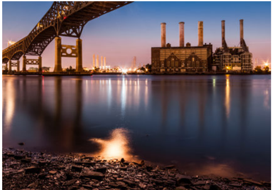
Kearny Power Station, Jersey City, NJ
