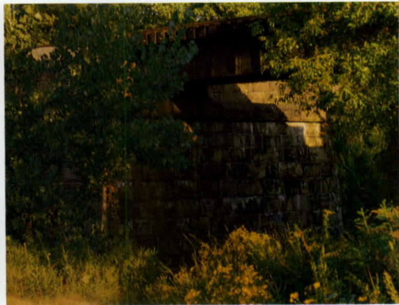
Railroad trestle over S. Branch Rahway river.
