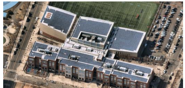
Figure 4. Non-residential behind the meter rooftop. Located at Central High School in Newark, NJ, this array totals 0.5 MW. Image source: Nearmap
