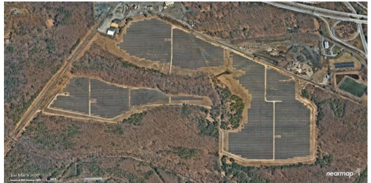
Figure 3. Grid supply solar PV. The largest grid supply solar array in the State; 28.5 MW ground mounted array at Earle Naval Base in Tinton Falls, NJ. Image source: Nearmap
