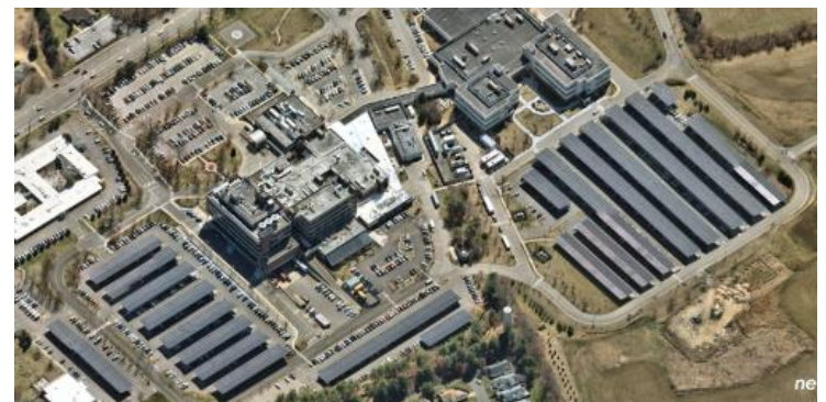
Figure 5. Non-residential behind the meter elevated carport array(s). Located at CentraState Medical Center in Freehold, NJ these arrays total more than 5 MW. Image source: Nearmap
