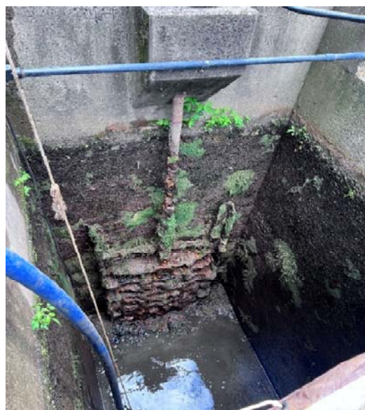
Original sluice gate in dewatered lock
