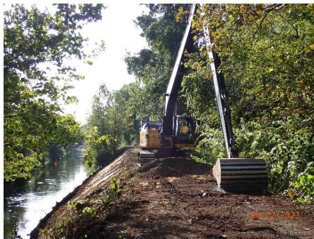
Restoration of the Canal embankment in Stockton
