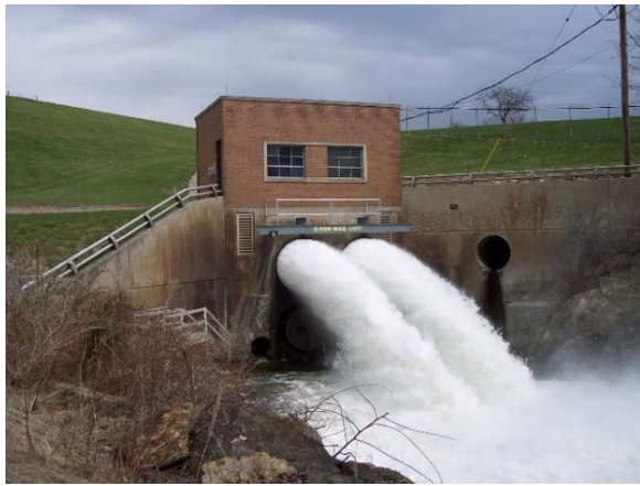
Spruce Run Reservoir's Outlet Vault
