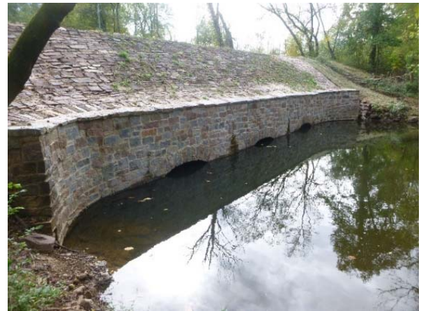
Rehabilitated outlet headwall at Six Mile Run Culvert
