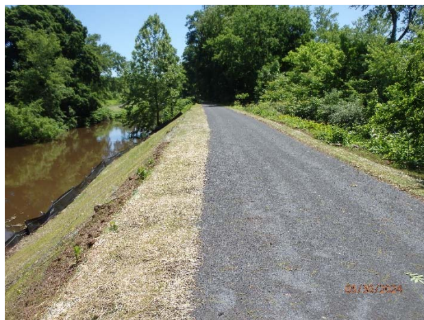
Restored Canal embankment in Stockton
