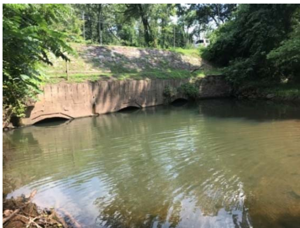
Outlet Headwall at Six Mile Run Culvert
