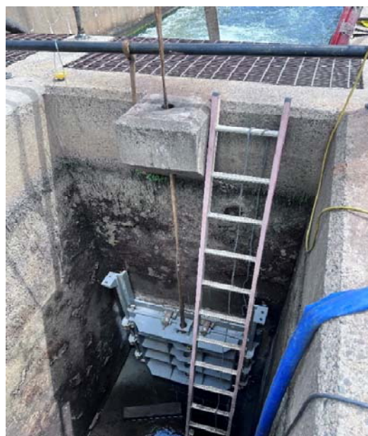
Replacement sluice gate
