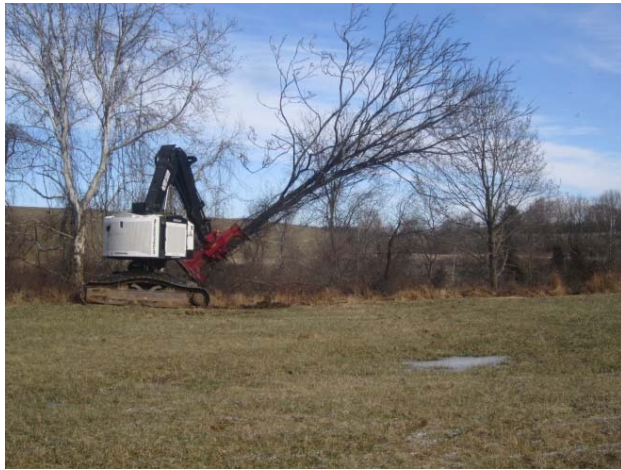
Tree clearing equipment at the spillway discharge channel
