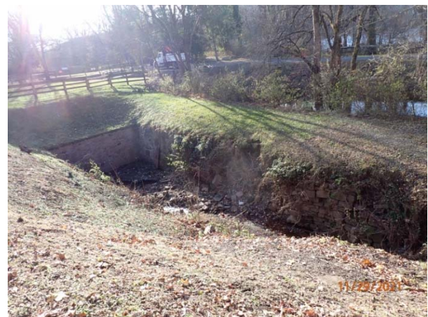
Existing condition of the Prallsville Culvert Pit.
