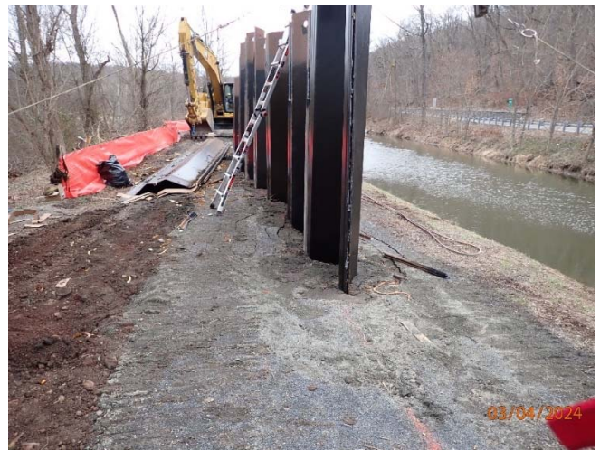
Steel sheets driven into Canal embankment
