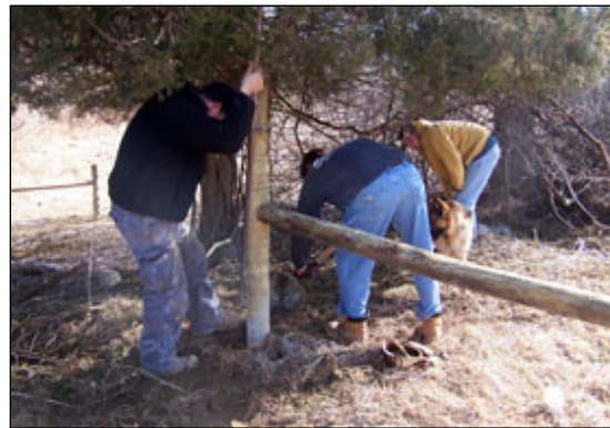
Fencing being installed at Howling Wolf Farm in Hope.
