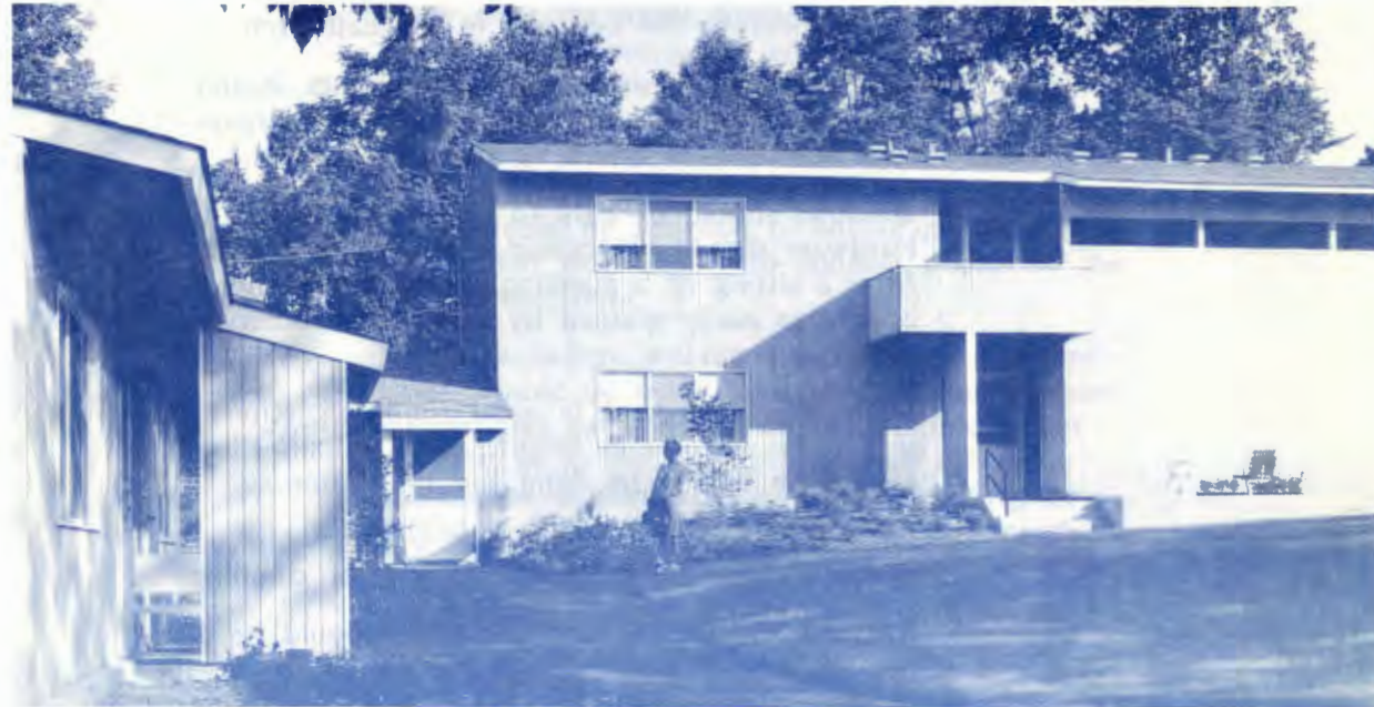
A site plan (top) was one of the first steps in the development of Lloyd Terrace (bottom), a 50-unit low-income housing development in Princeton.
