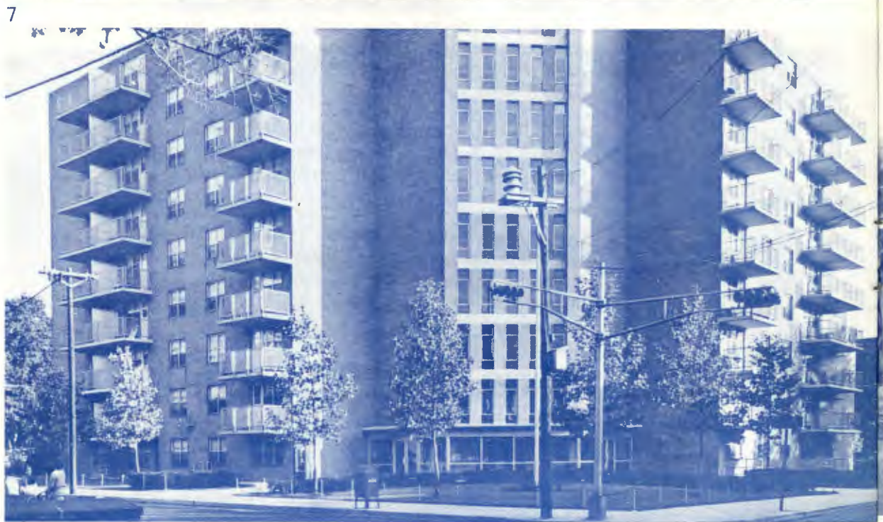
The 96-unit Nathan Barnert Homes (top) and the 100-unit Rev. William L. Griffin Homes (bottom) are low-rent housing developments in Paterson.
